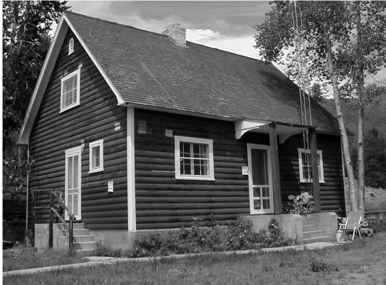
Dutch Joe Dwelling, one of two R4 Plan 8s on the forest. Note the boxed eaves and rake boards. Jim Bailey/USFS Photo
