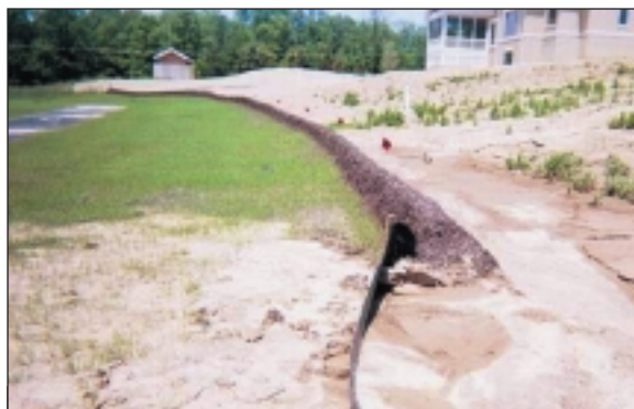
This filter berm made from compost demonstrates how well the organic material helps retain runoff in comparison to a typical silt fence in the lower portion of the photo.
