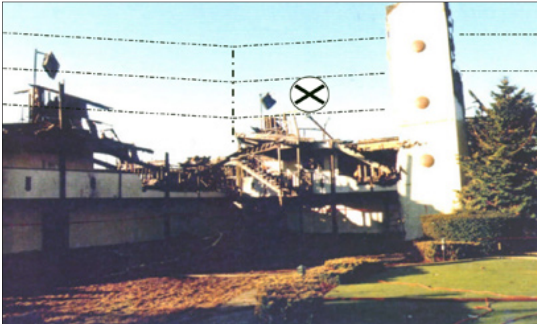
Photo 3. The view from the interior courtyard toward the SW corner. The X approximates the apartment of origin. Note the hose cabinets and piping still standing
