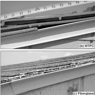
Figure 2—Side view of installed shingles: (a) western redcedar (WRC), (b) wood-thermoplastic composite (WTPC), and (c) fiberglass.
