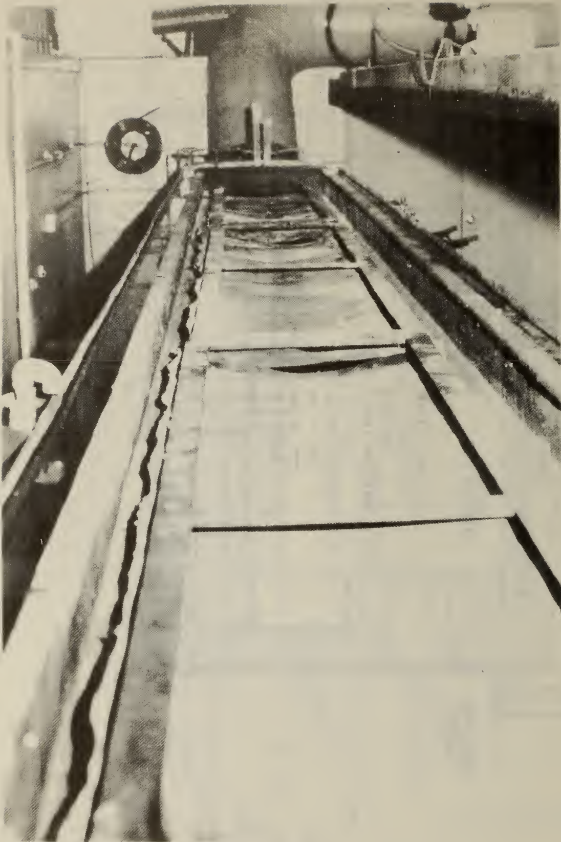
Figure 4. Screen wire test frames in place on tunnel ledges
