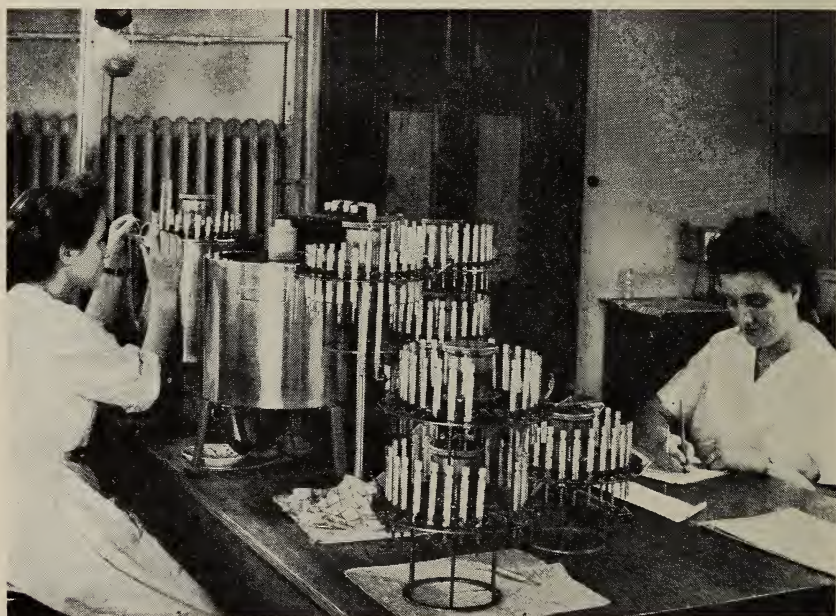
Official test of clinical thermometers by a Metrology Office.
