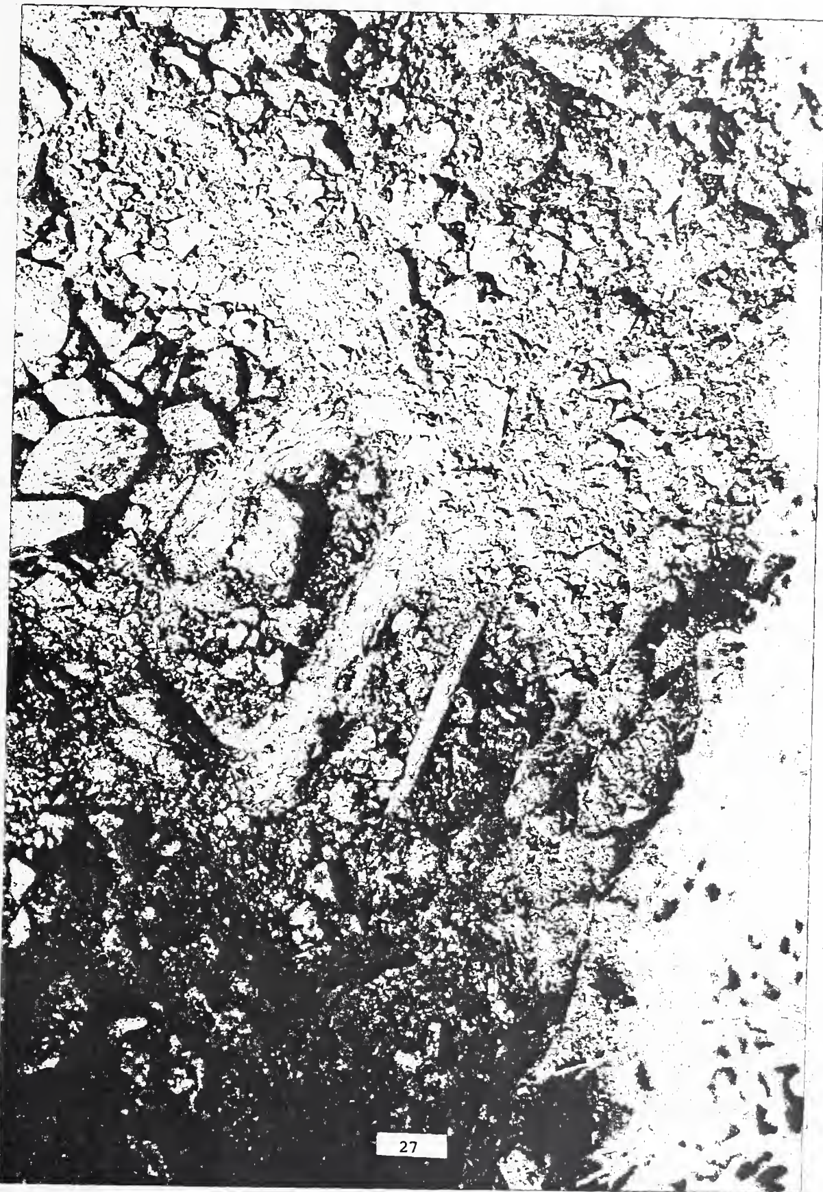
Figure 10. Rock rubble bed for water and sewer services at 4909.
