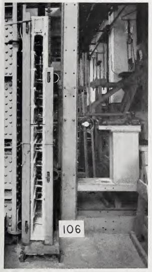
FIGURE 6.—Wall specimen BE-T1 under transverse load.
