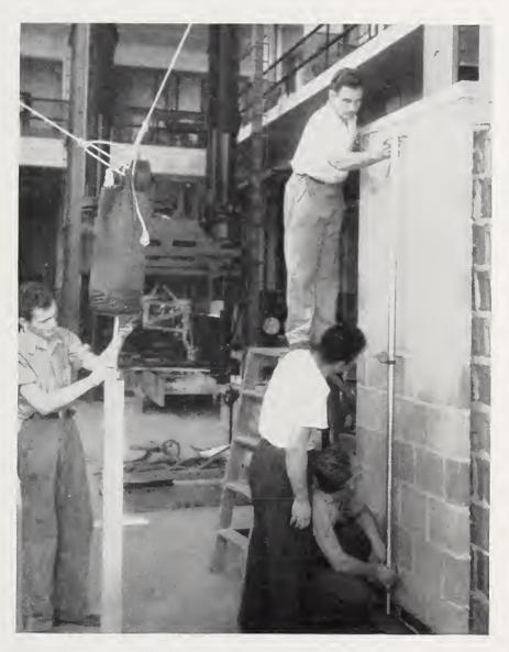
FIGURE 12.—Wall specimen BE-I1 during the impact test.
