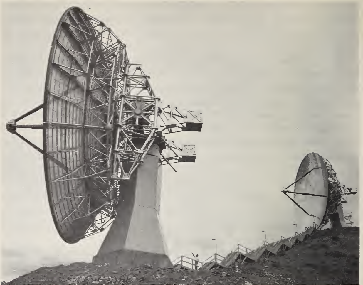
Two of the three 60-ft diameter paraboloidal antennas installed to make improved measurements of radio wave refraction in the earth's atmosphere (pages 5, 115).
