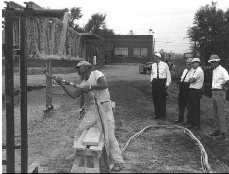
Figure 3 Demonstration of Monokote spray-on fireproofing circa 1967 at Laclede Steel Co. (Madison, Il.)
