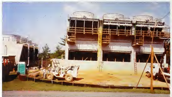
FIGURE 2. The new plume-abated cooling tower (right) nears completion. It will replace the lower capacity and less efficient system that had no abatement ability (left).
