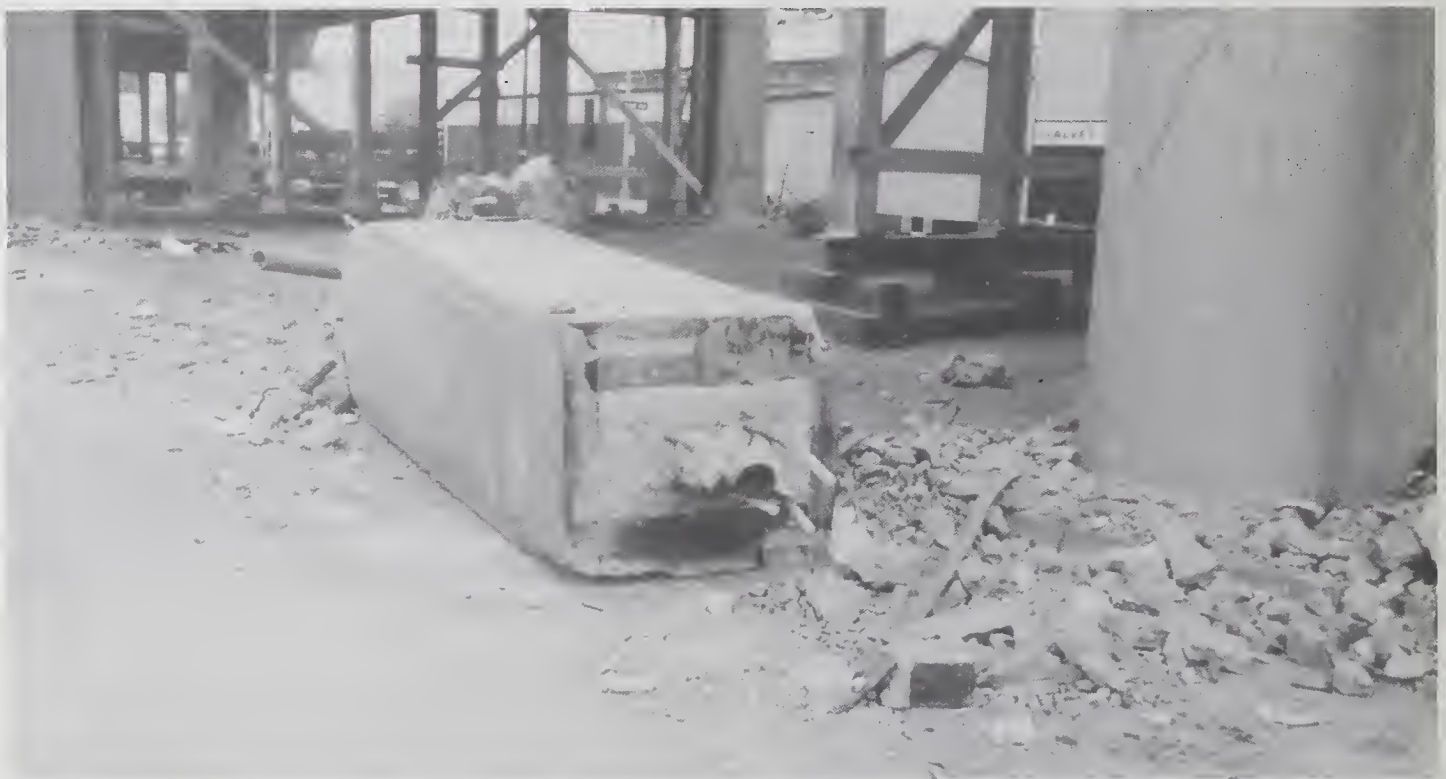
Figure 5.6.35 Detail of the bottom of the two-hinged column that was ejected from the west side of Bent 71 showing central pipe used to drain the upper road deck and the 4-#10 dowel bars used to transfer shear across the hinge.
