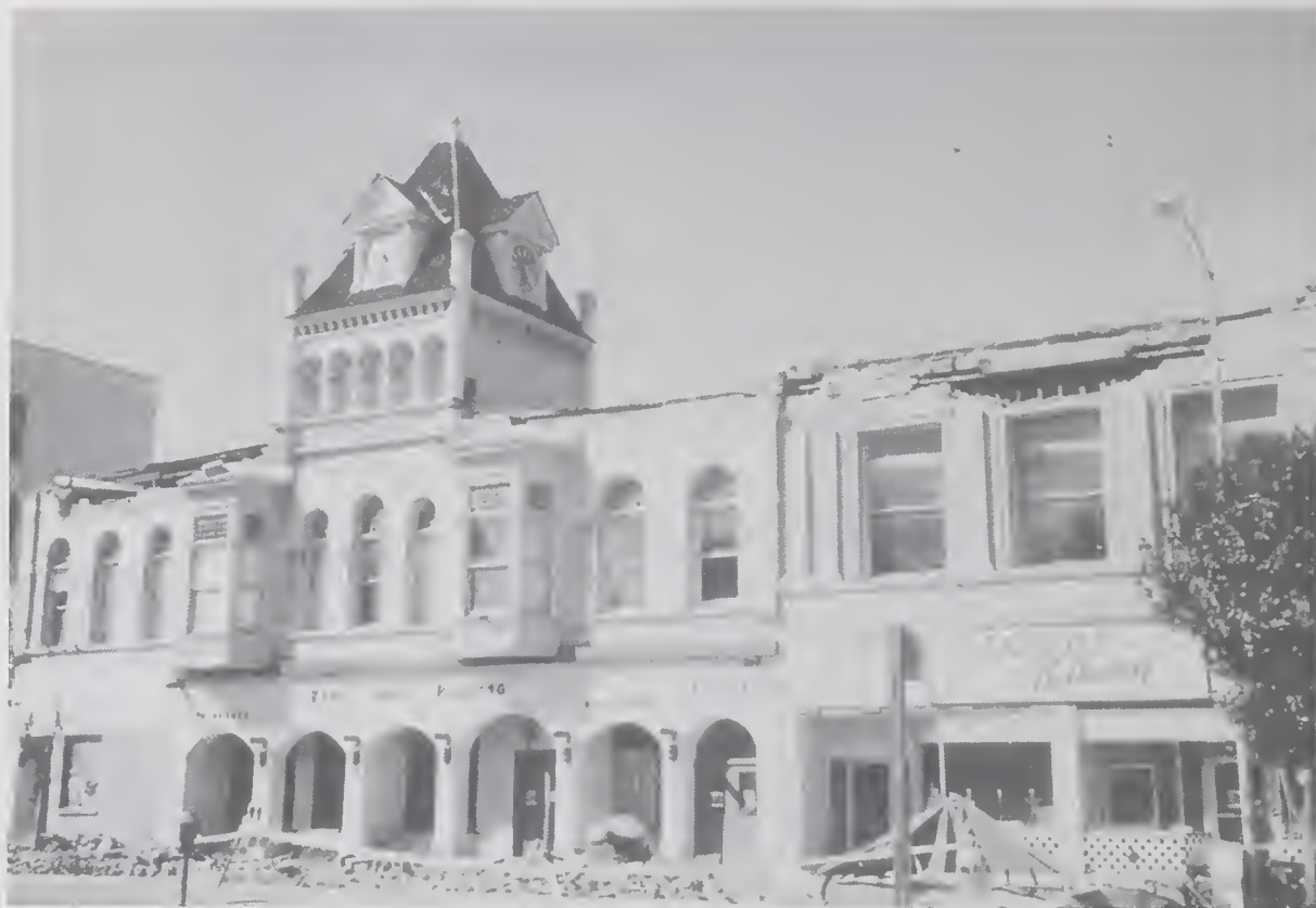
Figure 4.4.5 Falling brick from this old masonry building in Watsonville caused one death.
