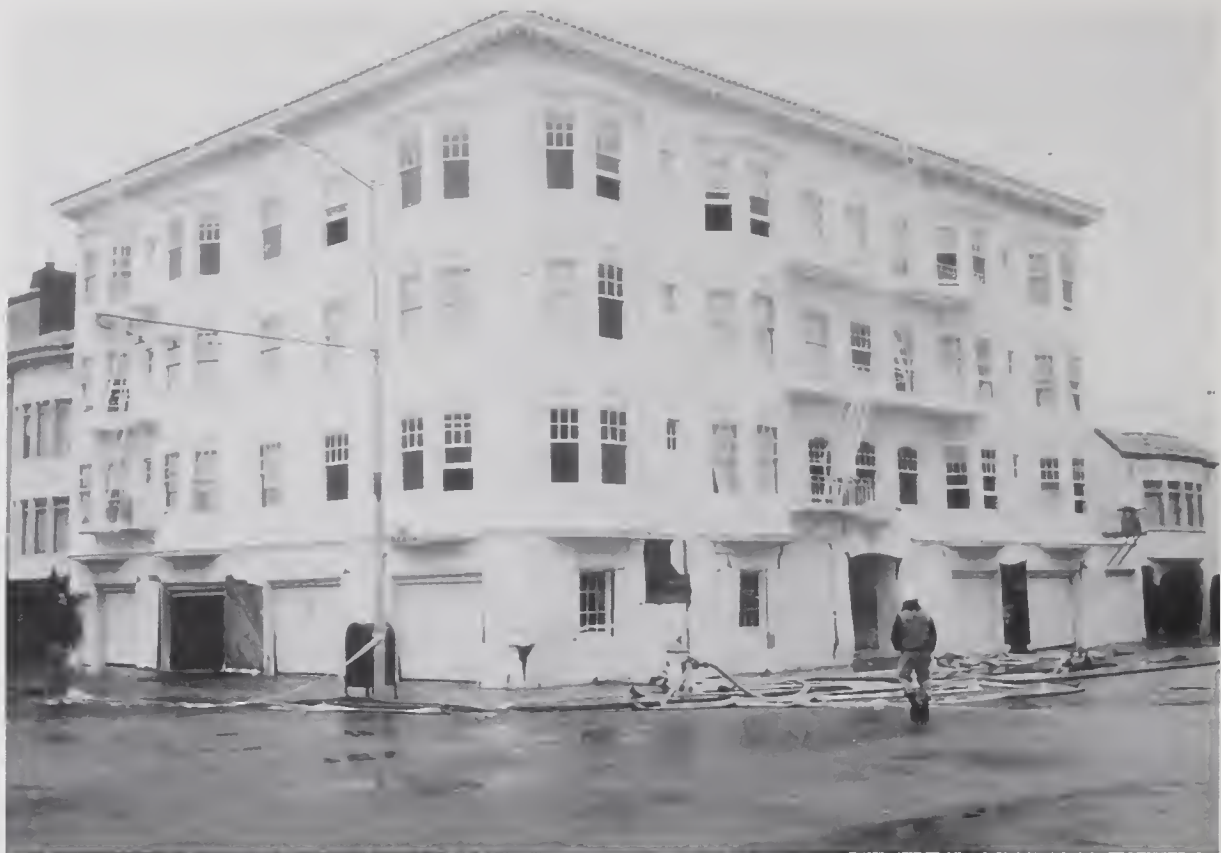
Figure 4.2.12 Example of four-story building with multiple garages in the first story (location #6).
