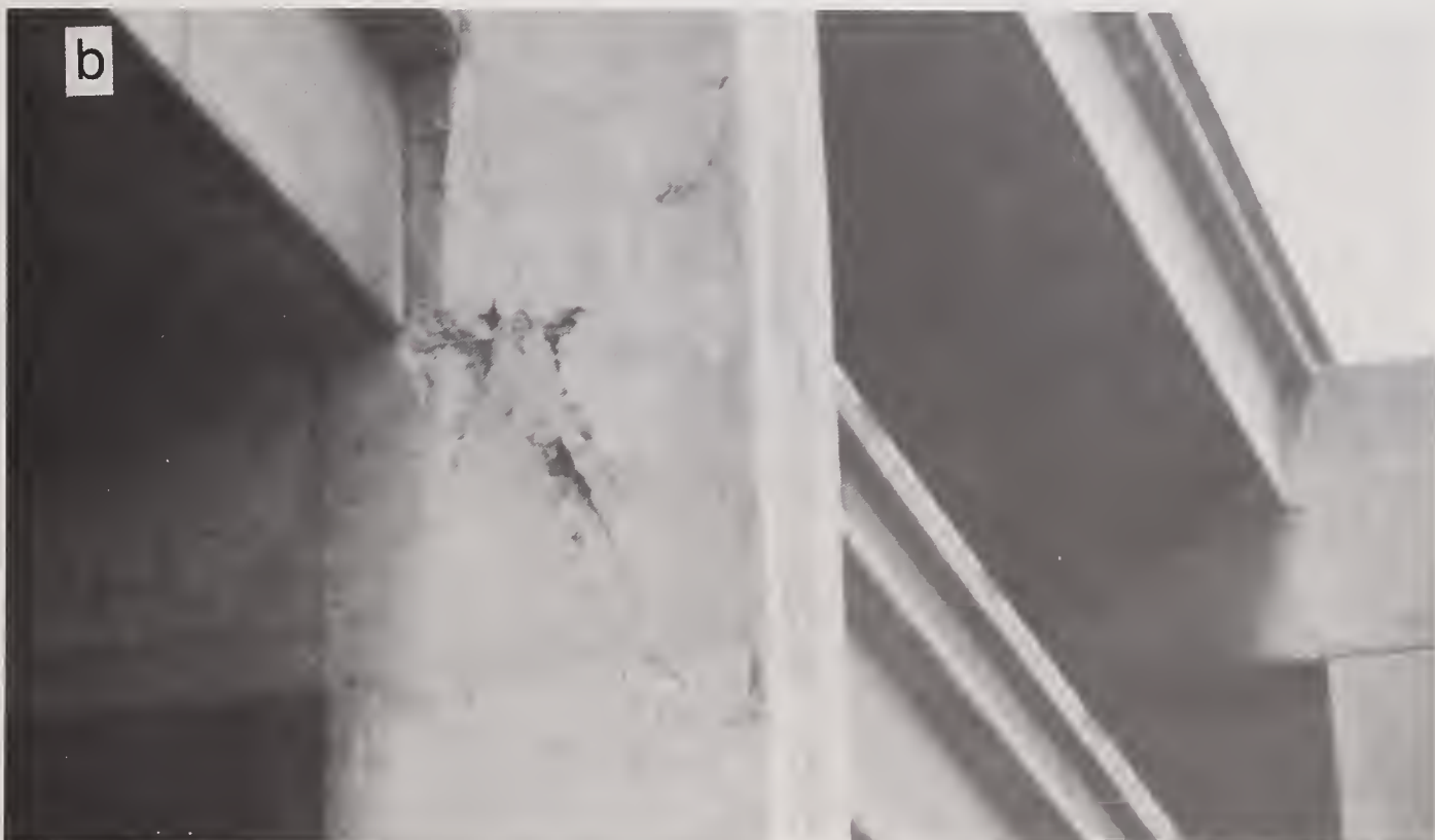
Figure 5.10.5 (a) Close-up view of west side of Bent 78 showing diagonal cracking in joint and vertical cracking at girder-column boundary; (b) close-up view of east side of Bent 79 showing diagonal cracking in joint.
