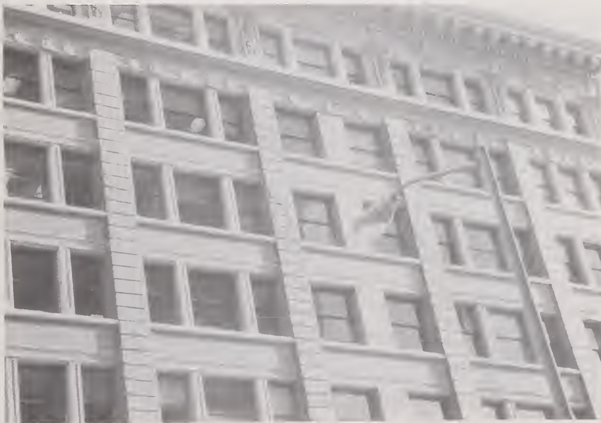
Figure 4.2.32 Example of damage to masonry cladding of Wells Fargo Bank building (location #7).
