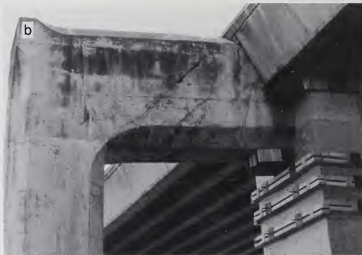
Figure 5.9.15 (a) Bent 32 supporting I-280 at Sixth St. exit ramp and (b) close-up of girder showing diagonal cracking.
