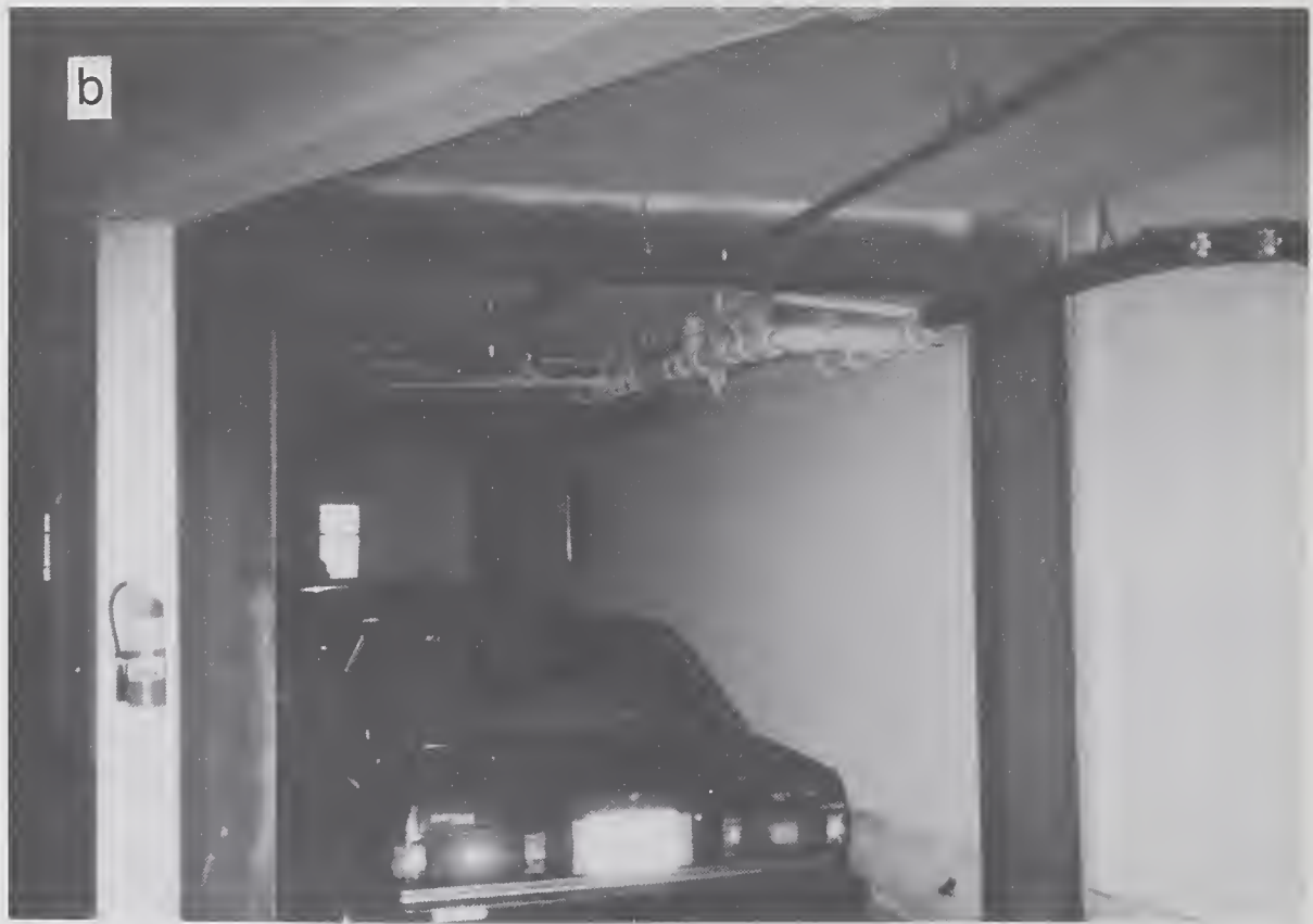
Figure 4.2.22 (a) An undamaged, three-story building (location #8) and (b) view of the moment-resting frame used for retrofitting.
