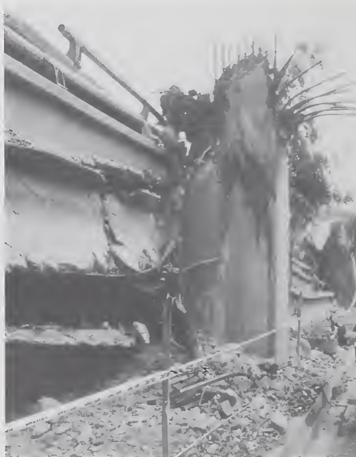
Figure 5.6.38 The section of Cypress Structure between Bents 104 and 106 was the only location in which both upper and lower bent frames failed.
