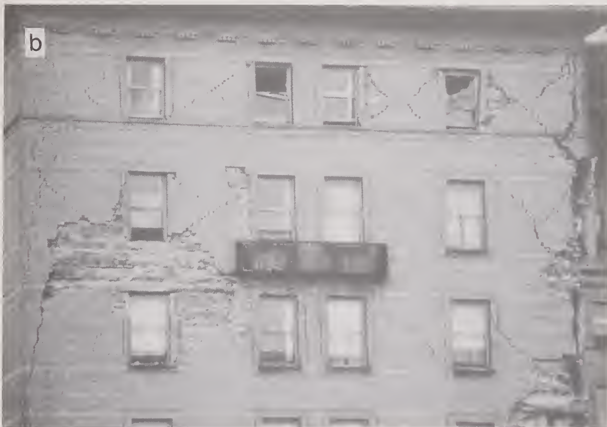
Figure 4.3.3 Oakland Hotel: (a) View of west wing and (b) close-up view of damaged masonry infill (location #6).
