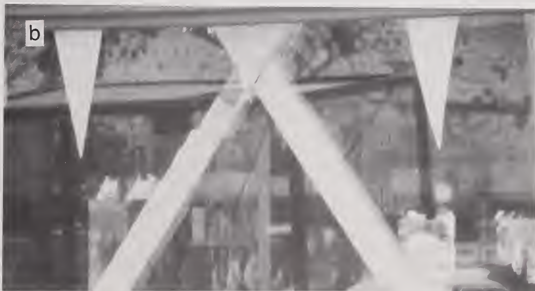
Figure 4.2.29 (a) The historic DeBernardi warehouse building showing the bracing added during seismic retrofitting; (b) close-up view of the bracing showing damage caused by earthquake.
