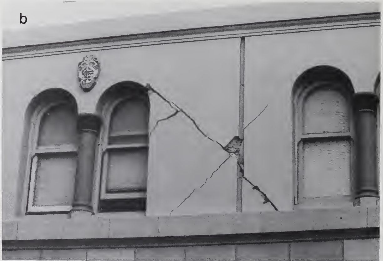
Figure 4.4.11 (a) Seven-story, reinforced concrete building suffered severe cracking; (b) Close-up view of damage to second-story walls.
