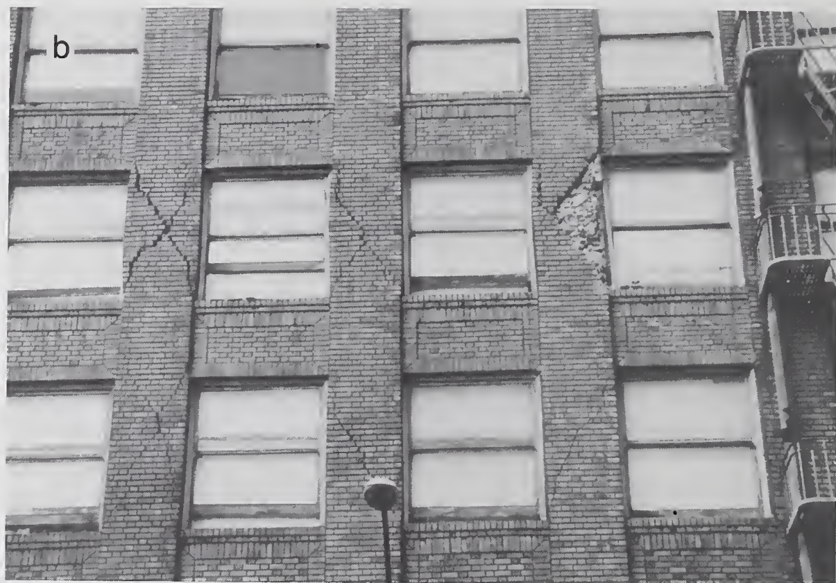
Figure 4.3.2 Dalziel apartment building: (a) overall appearance and (b) close-up view of cracking in masonry piers (location #1).
