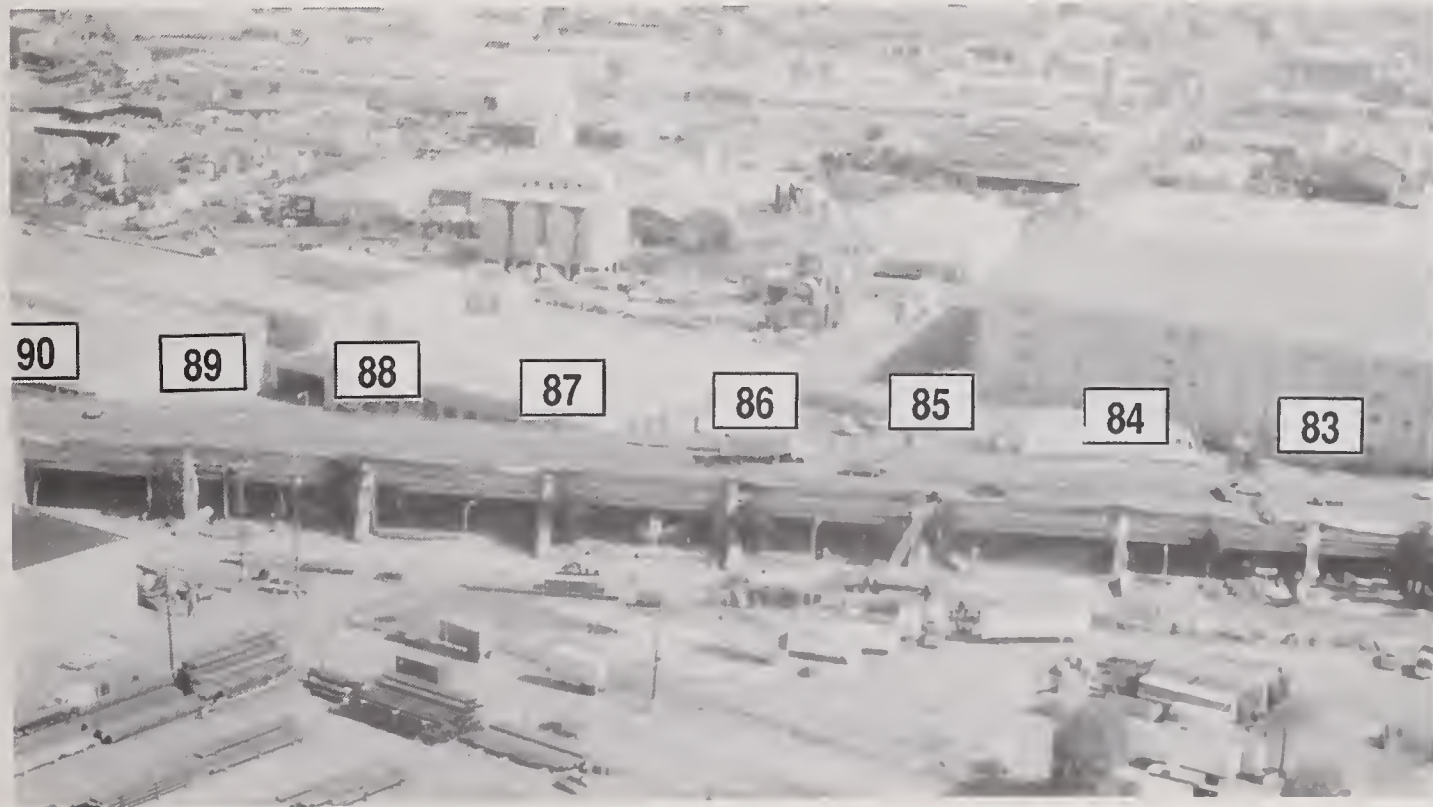
Figure 5.6.17 Aerial photo looking east to the collapsed portion of Cypress Structure between Bents 83-90.
