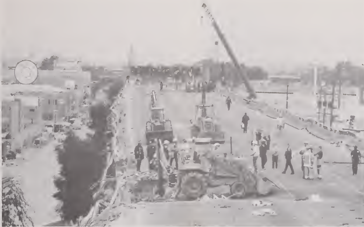
Figure 5.6.24 View of the upper deck of Cypress Structure looking north of Bent 80. This photo illustrates the negligible lateral displacement of the upper deck relative to the lower deck during the collapse.
