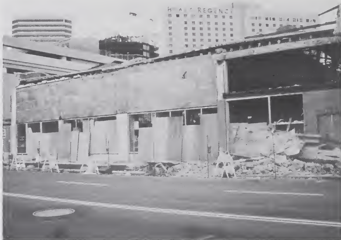
Figure 4.3.5 Extensive damage occurred to a two-story unreinforced masonry building built in 1917 (location #3).
