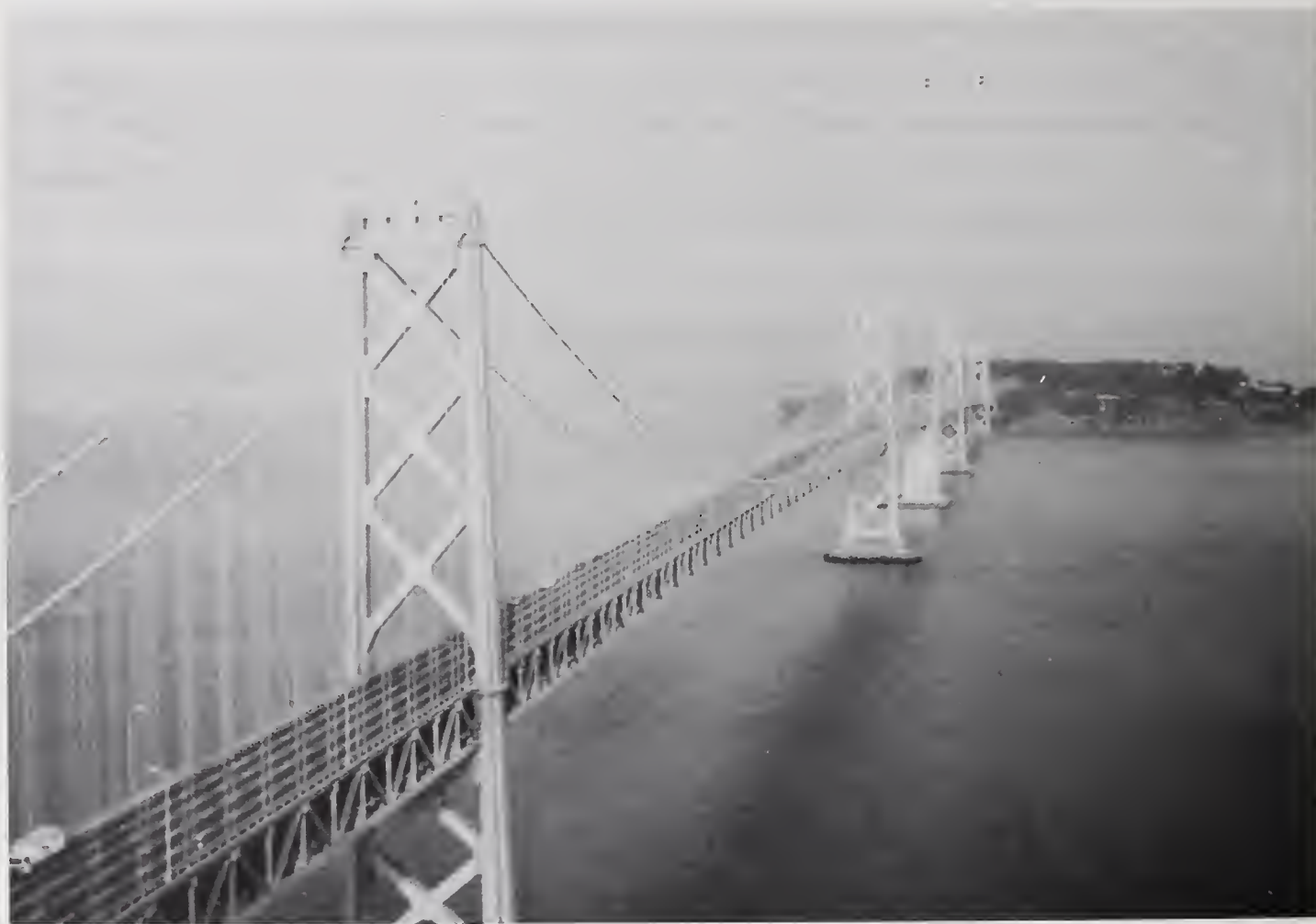
Figure 5.7.1 View looking east from San Francisco to Yerba Buena Island showing the two main suspension spans for the Bay Bridge. No damage was detected in this section.
