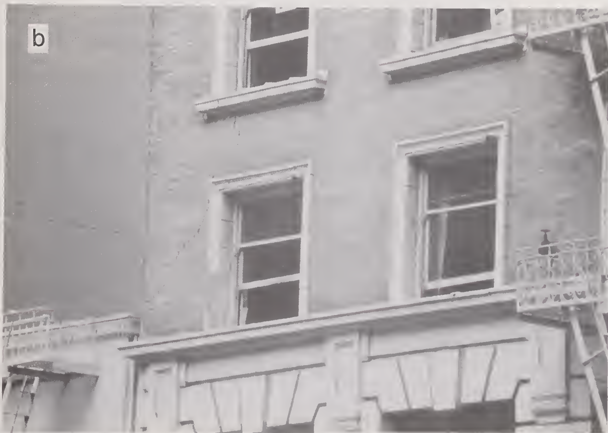
Figure 4.2.27 (a) Severely damaged Marine Building at corner of Front St. and California St.; (b) Close-up view of the northwest corner showing severity of cracking.
