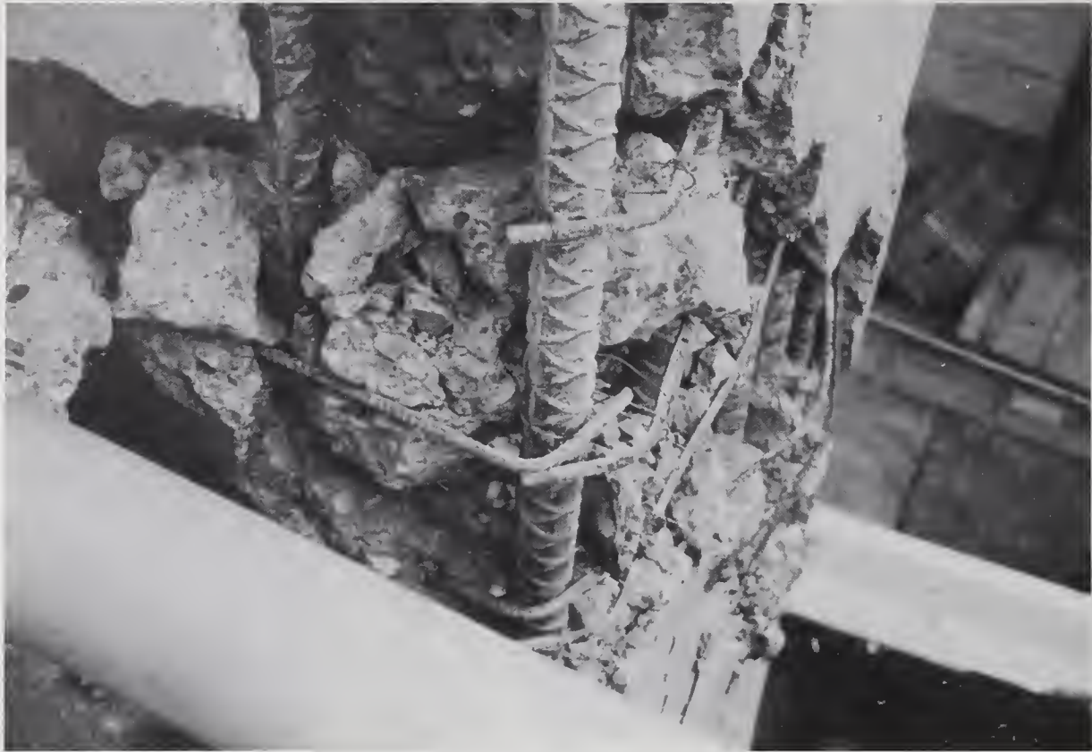
Figure 5.9.9 Close-up view of the failure zone of Bent 51, showing anchorage failure of ties.
