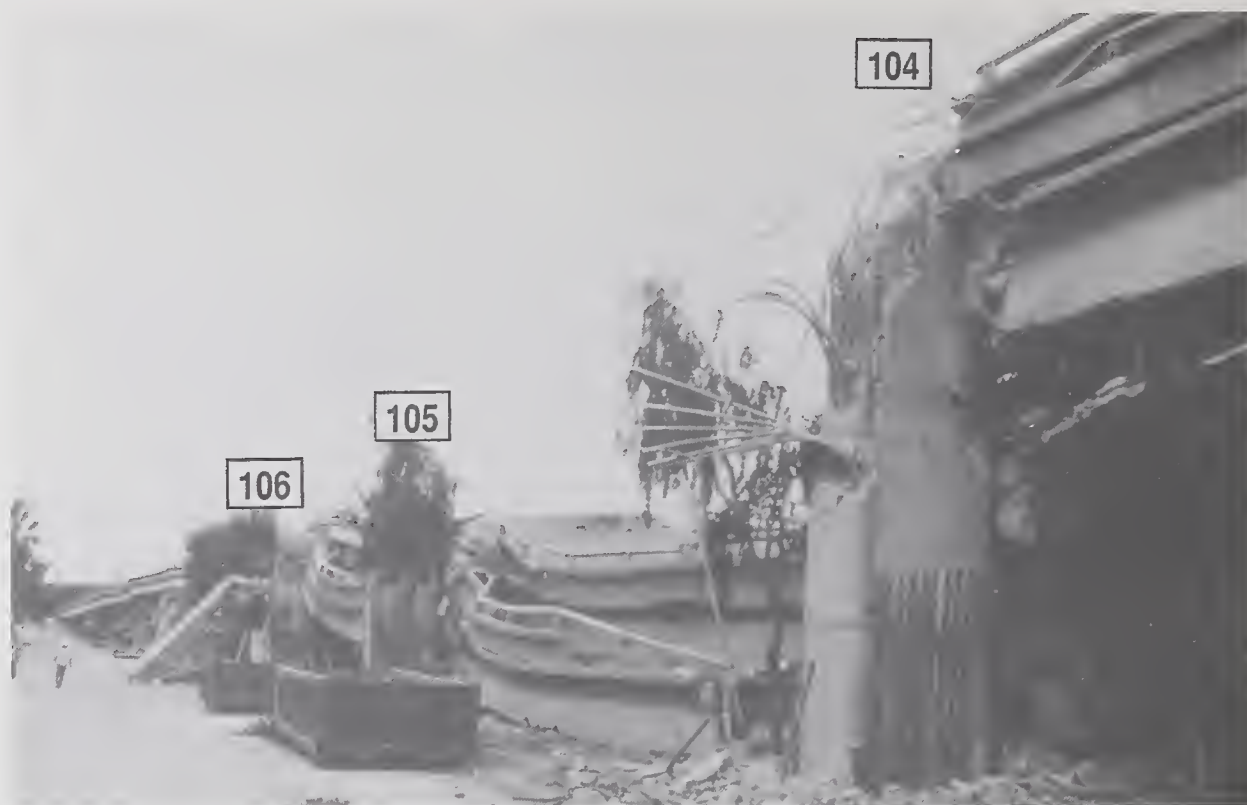
Figure 5.6.38 The section of Cypress Structure between Bents 104 and 106 was the only location in which both upper and lower bent frames failed.
