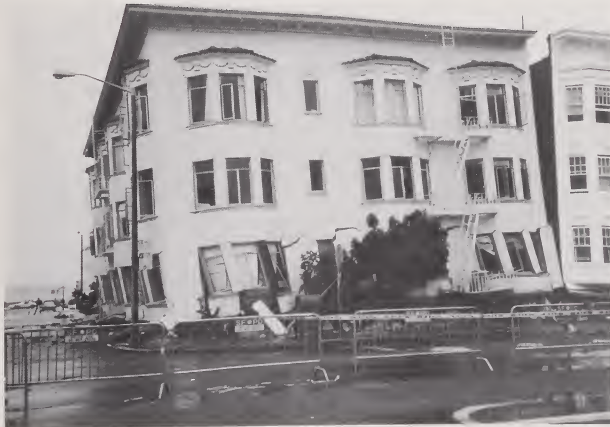
Figure 4.2.7 Two four-story buildings which suffered total collapse of their first stories (location #14).
