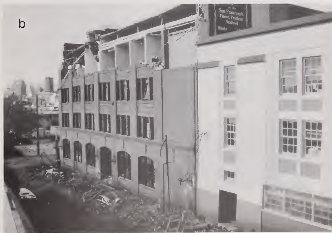
Figure 4.2.34 (a) Damage to upper story of unreinforced masonry building on Bluxome St. (location #8); (b) damage to the southwestern wall which resulted in the death of six persons.
