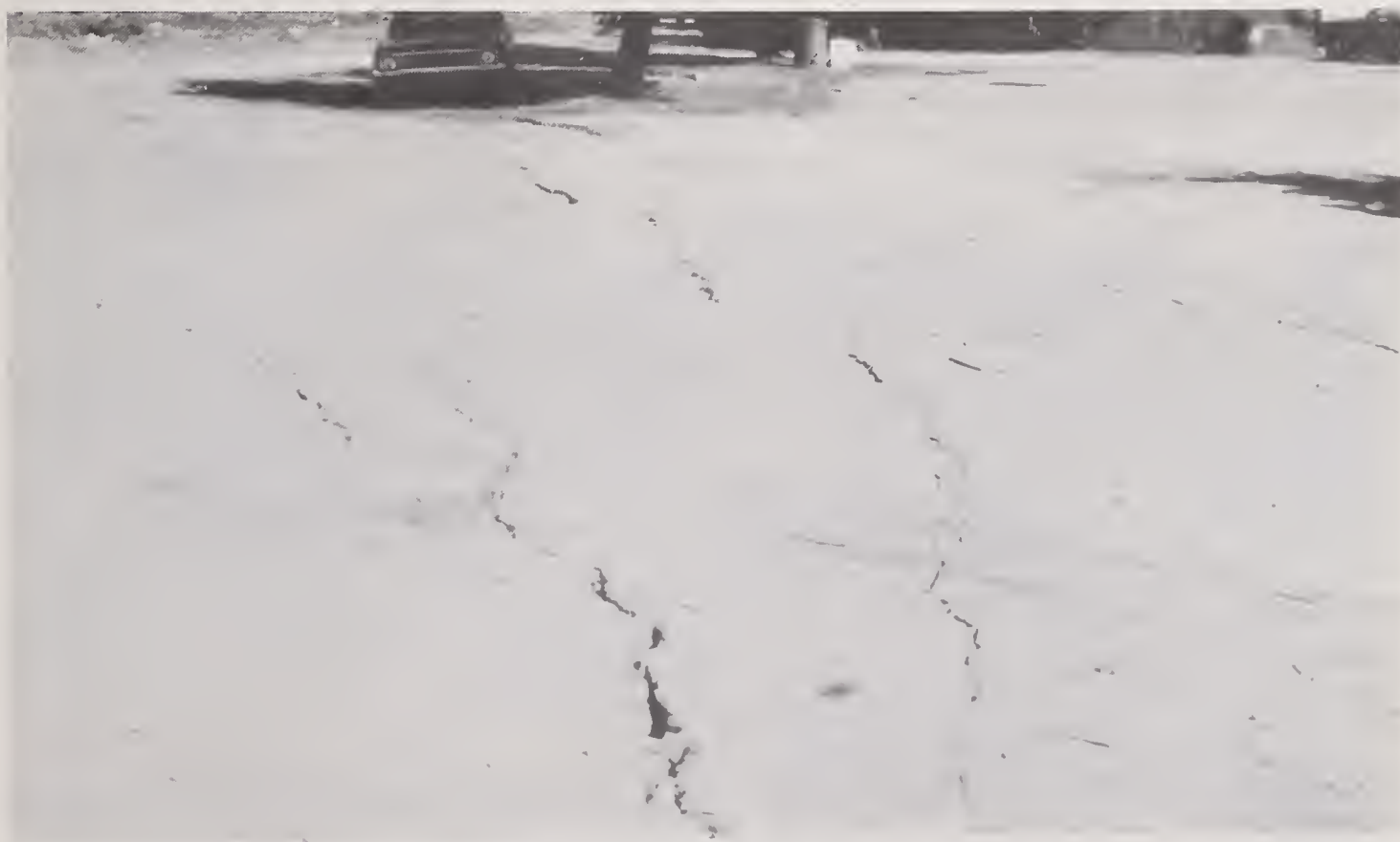
Figure 3.3.9 Tension cracks behind Pajaro River levee.
