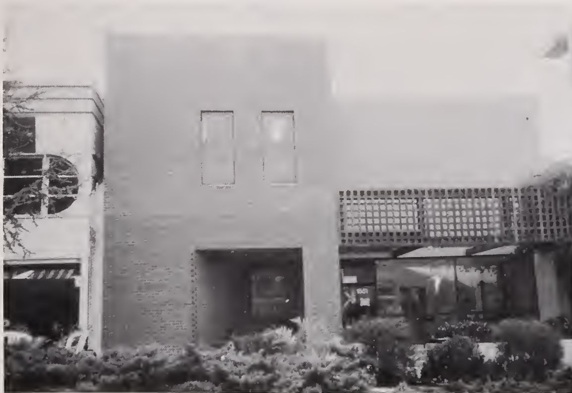
Figure 4.4.9 Modern reinforced masonry structure which was undamaged; building on the left suffered roof failure causing two deaths (location #1).
