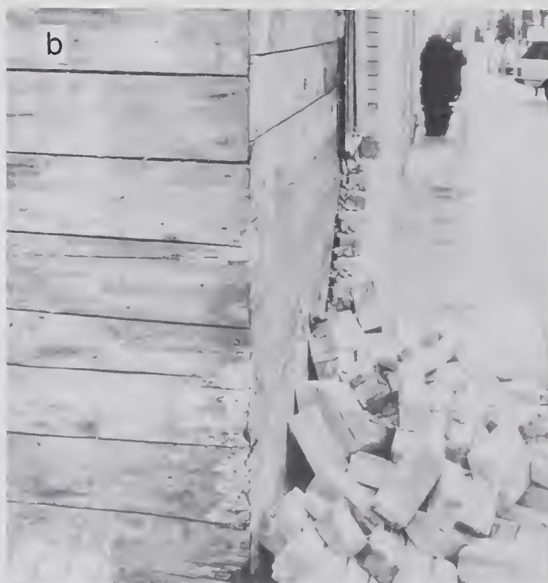
Figure 4.2.19 (a) Example of building with failure of brick masonry facade (location #12) and (b) close-up view of corner showing damaged wood and lack of anchorage to the masonry.
