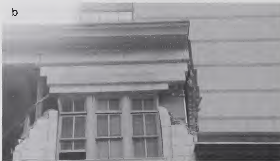
Figure 4.2.28 (a) Damage to the southeastern corner of the Golden State Bank Building; (b) Close-up view of the northeastern corner; damage was likely caused by pounding against the adjacent building.
