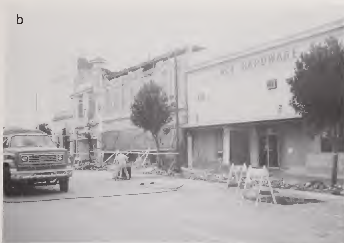
Figure 4.4.4 (a) Failure of wood-framed building with masonry walls and multiple opening in first story (Los Gatos); (b) typical damage to parapets and storefront windows (Watsonville).
