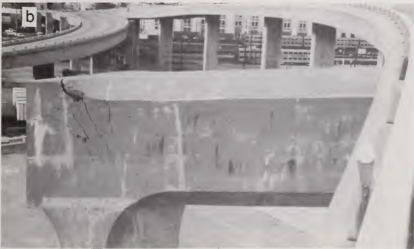
Figure 5.9.14 Damage to girder supporting exit ramp: (a) eastern portion and (b) western portion.
