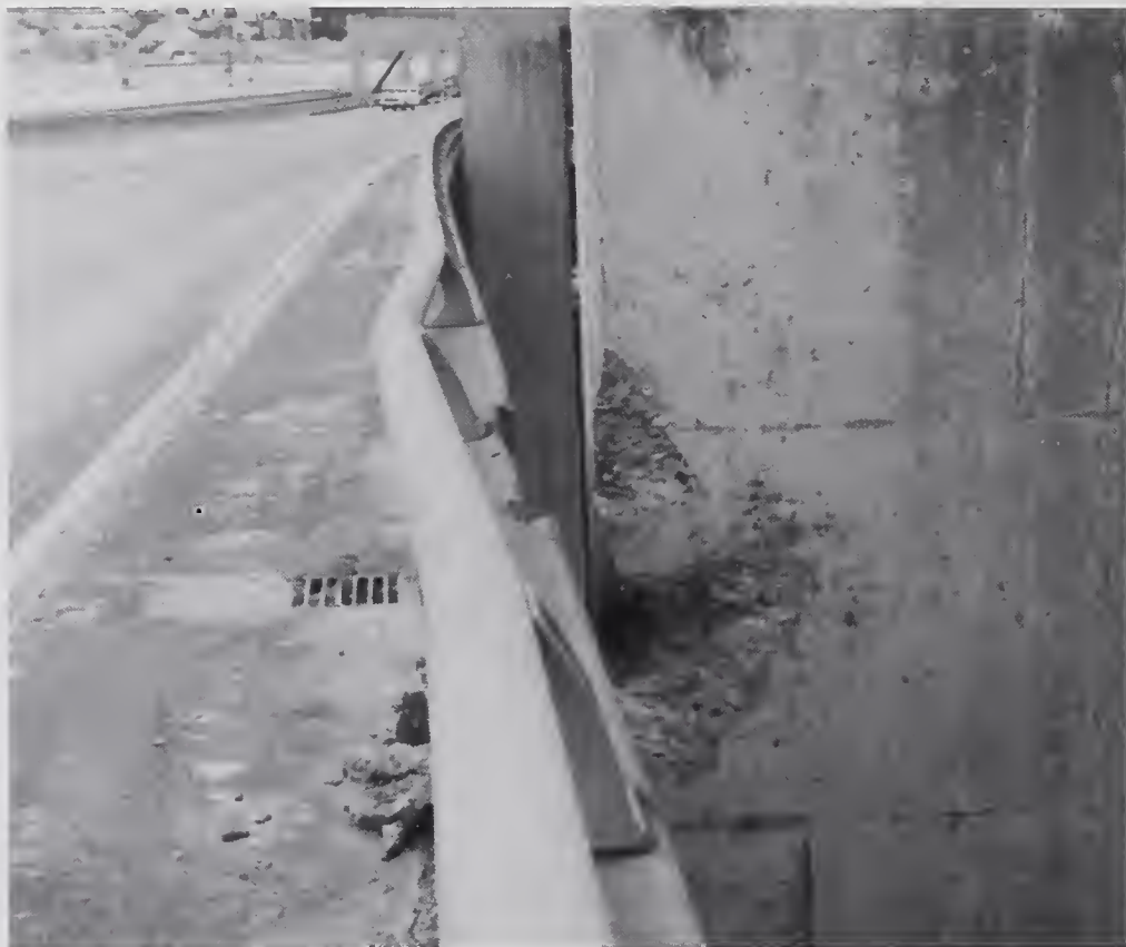
Figure 5.9.10 Pounding damage at I-280 south of Army Street.
