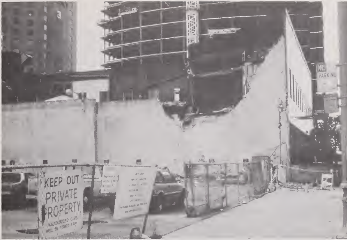
Figure 4.3.6 Collapse of unreinforced masonry wall crushed vehicles in adjacent parking lot (location #5). In background is a steel-framed building under construction which sustained damage.
