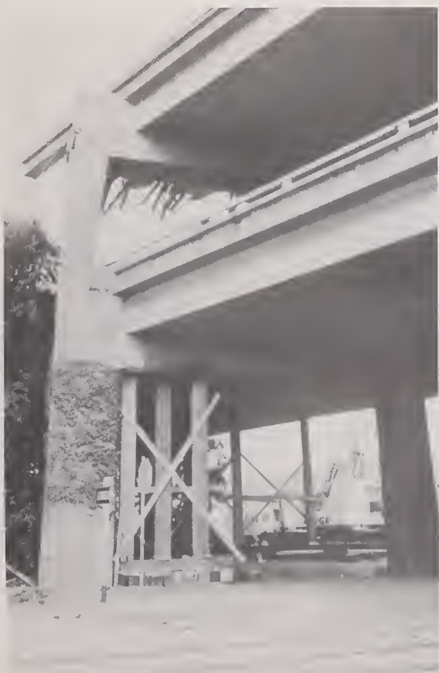
Figure 5.6.36 View looking west towards Bents 96 and 97 which supported the only segment of the upper deck to remain standing between Bents 62 and 113.
