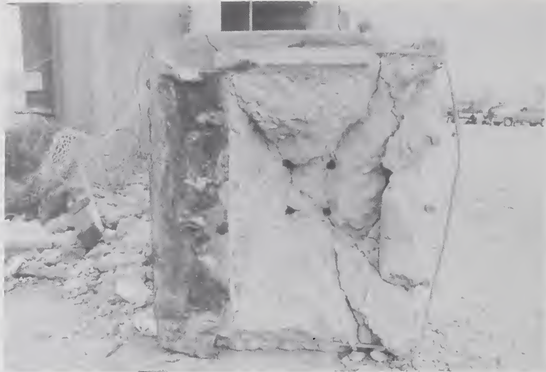
Figure 5.6.34 Detail of the base of the two-hinged column that was ejected from the west side of Bent 72. The 4-#10 dowel bars which passed through the center of the shear key have been pulled free.
