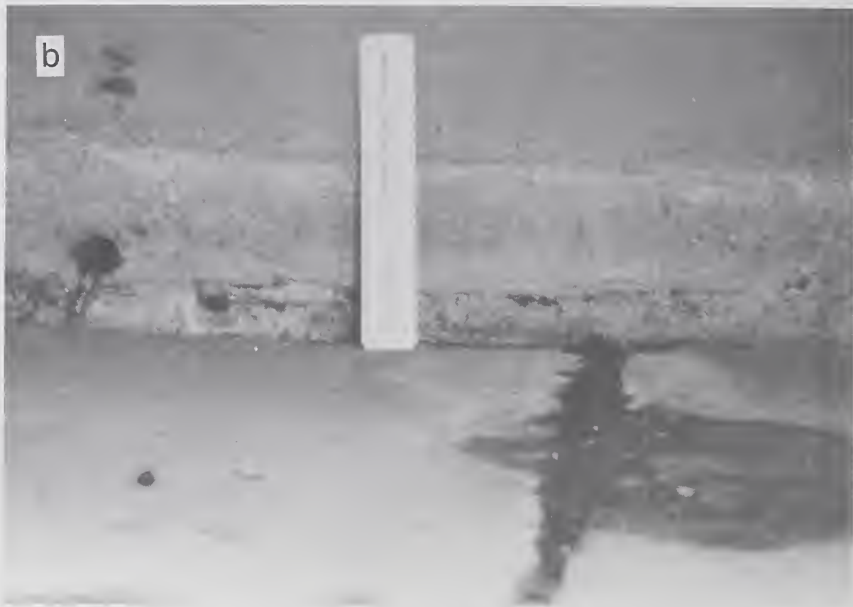
Figure 4.2.26 (a) Sidewalk showing distortions due to differential settlements, and (b) close-up view of intersection of sidewalk with retaining wall showing magnitude of differential movement.
