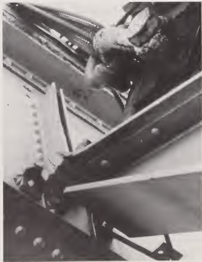
Figure 5.7.7 Close-up of the western girder seats for the lower road deck at Pier E-9. Lack of significant damage to these seats, and to those supporting the upper road deck, indicates that both upper and lower segments moved eastward by an amount sufficient to permit both to slide off the western seats and drop simultaneously.
