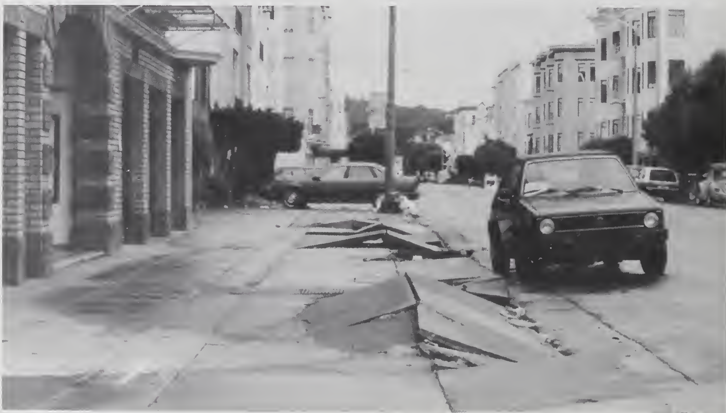
Figure 3.3.4 Typical liquefaction damage in the Marina District of San Francisco.
