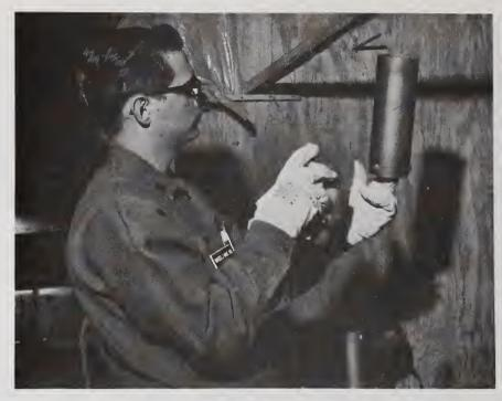
Figure 2. Priming a fuel sleeve.
