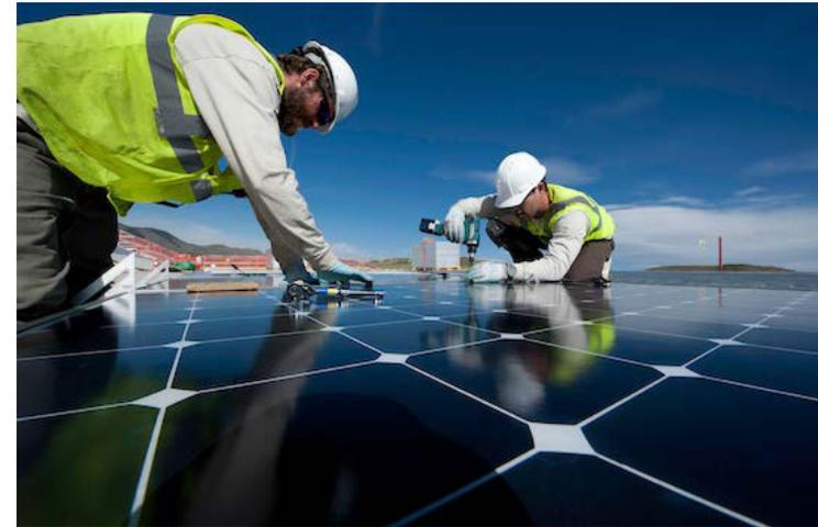
install one of the 3,632 solar modules on NREL's parking garage. The garage can produce up to 1.15 megawatts Photo by Dennis Schroeder / NREL 21487
