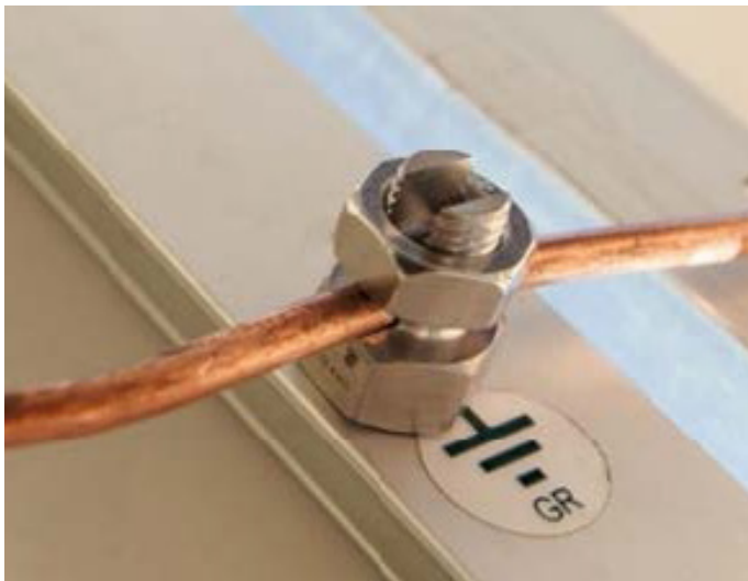
Figure 1: Common ESD/ordnance grounding point
