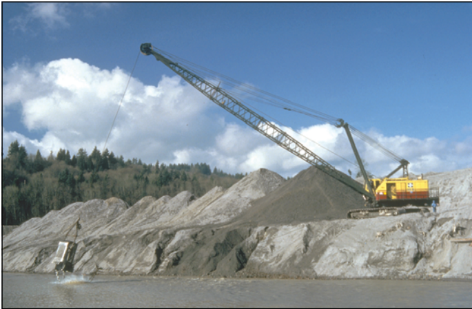
Figure 24. Photograph of U.S. Army Corps of Engineers dredging the Toutle River after the 1980 eruption of Mount St. Helens, Washington. Dredging was also necessary in the Cowlitz and Columbia Rivers. By 1987, enough volcanic debris to pave a 12-lane highway from New York City to San Francisco had been removed from these three rivers. Photograph by L. Topinka, U.S. Geological Survey.
