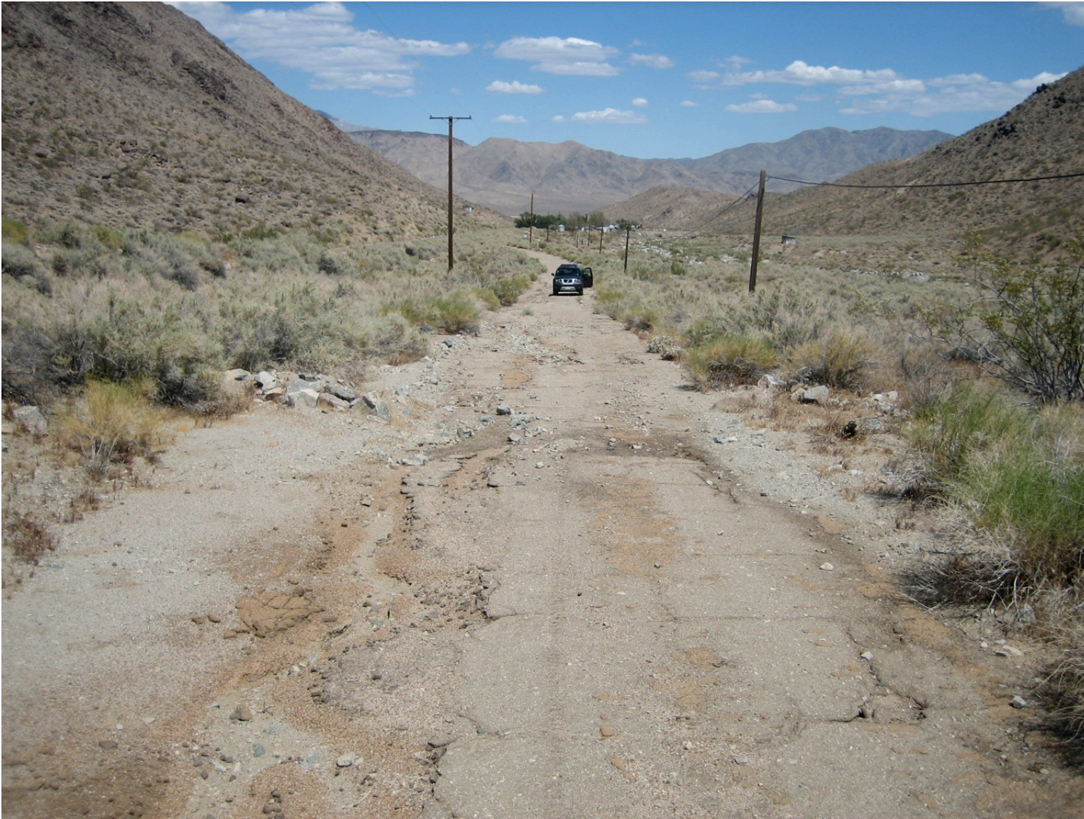
Figure 9. Tailings used in construction of the old road in the central part of Homewood Canyon. Sample sites T5 –T9 shown in figure 5.
