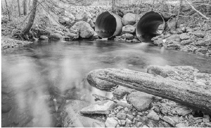
Roaring Brook culvert prior to replacement. At lower flows this culvert outlet was perched above the water surface, creating a barrier to the movement of fish. The stream was constricted by the pipes' combined span of 12 feet, which caused debris buildup and localized flooding.
