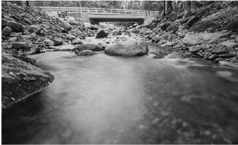
Roaring Brook culvert replacement: With a width of 35 feet, the new culvert—an open-bottom concrete box with a natural streambed—allows the stream to pass freely underneath, opening six miles of upstream habitat for fish and designed to withstand high water flows.
