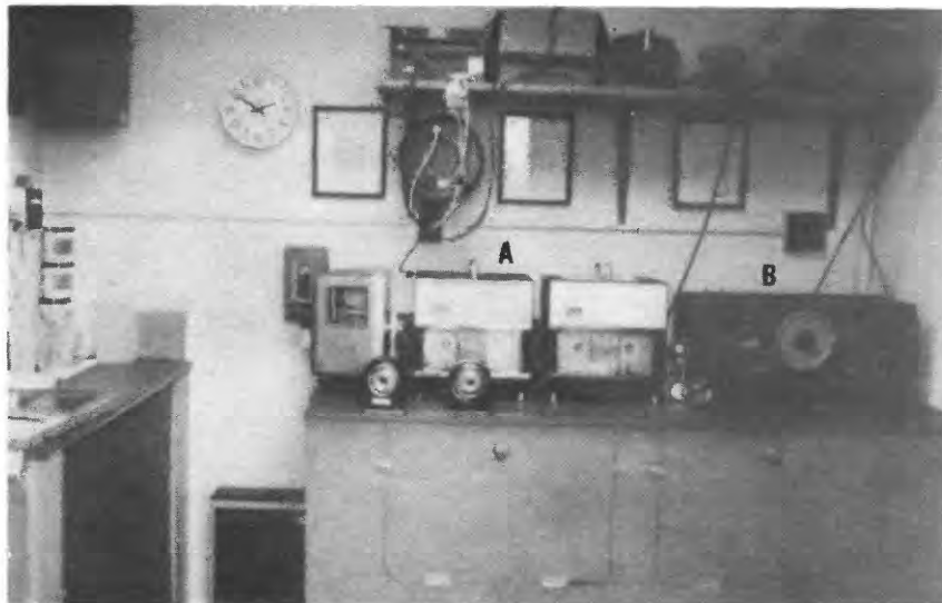
Figure 6.--Susquehanna River at Harrisburg, Pa. gaging station equipped with (A) analog digital stage recorder, and (B) a continuous strip- chart recorder.
