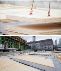
Construction of ARBORA complex with 435 residential units using massive timber in Montreal, Canada. Foto credit: Nordic Structures.
