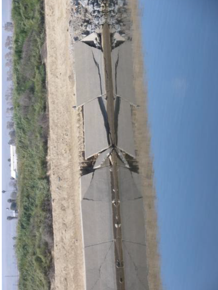
Figure 1. Damage to water infrastructure: Subsidence along the Delta-Mendota Canal
