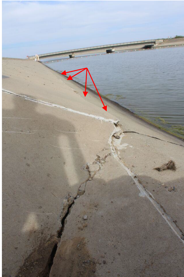
Figure 2. Damage to water infrastructure: A photo of subsidence along the California Aqueduct. The crack at the bottom of the photo is about 5 feet long and has caused the entire side of the canal to cave inwards. You can also see a crack developing that runs the length of canal (highlighted by arrows).
