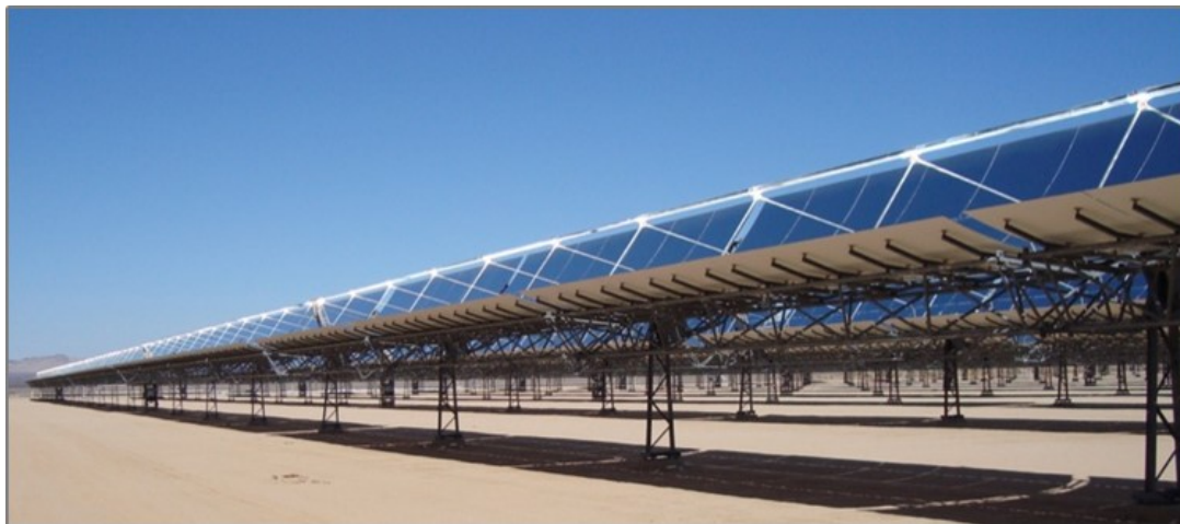
Figure 2: Parabolic reflectors with receivers at their focal line.
