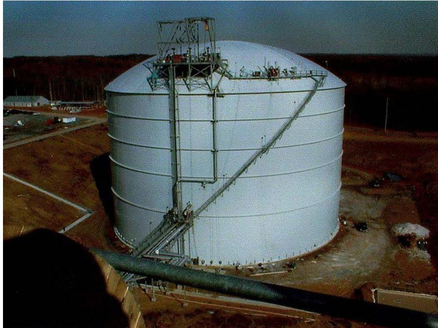
**Figure 7. Example of Large Cryogenic Storage Tank for Liquefied Natural Gas (public domain image courtesy of ferc.gov)**
