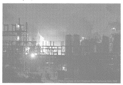
**Figure 3**: Equipment destruction along the trajectory of the residue treater vessel; the deformed shell of the vessel is visible at the center of the photograph.
