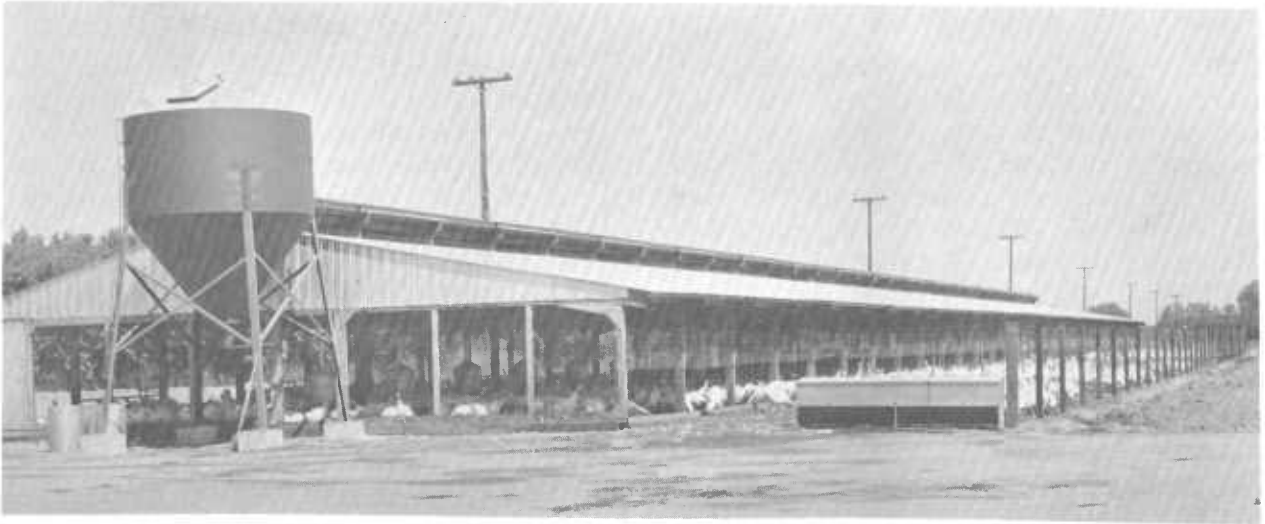
Figure 26. —Pole-type, 40- by 300-foot, semiconfinement rearing shelter with a 20-foot concrete porch (apron) along south side. Capacity of unit, including porch, is about 3,700 heavy-breed turkeys. Note full-length roof ventilator. (Photo from Turkey World, Mt. Morris, Ill. 61054.)
