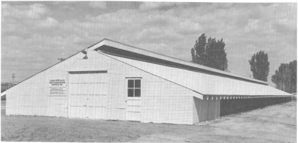
Figure 27. —Pole-type house for turkeys with full-length ventilation opening in roof facing away from prevailing winds. Plans may be obtained from Colorado State University, Fort Collins, Colo. 80521. (Photo from Colorado State University.)
