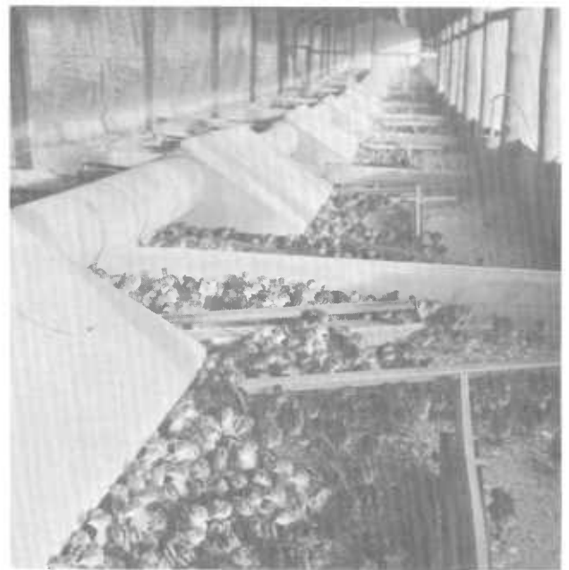
Figure 14. —Thermostatically controlled hot-air brooding system. Heat is furnished by furnace and is circulated through brooding units by fans. (Photo from Turkey World, Mt. Morris, Ill. 61054.)
