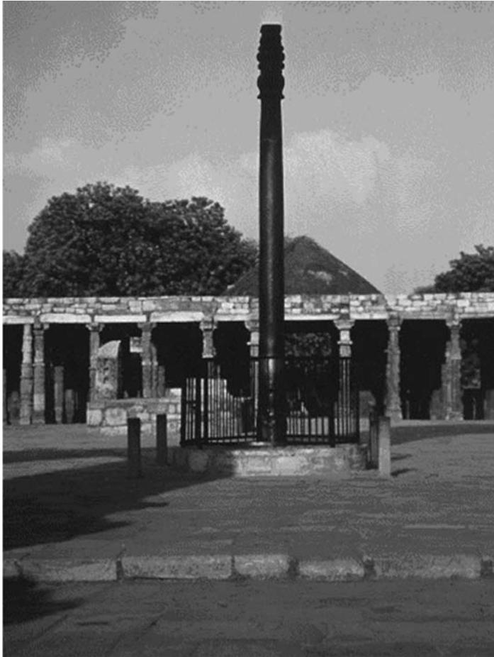
**Figure 48.** The corrosion-resistant iron pillar at Delhi, India (Balasubramaniam, 2000, fig. 1).
