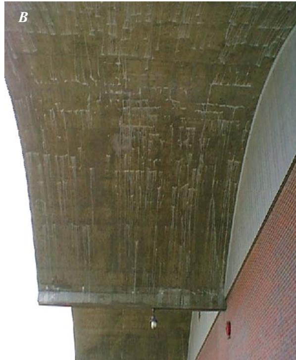
**Figure 59.** (A) Building 810 on the Denver Federal Center, Colorado, and (B) a closeup of the underside of the roof over a loading dock. Water has seeped through minor fractures in the concrete and flowed along the curvature of the roof rather than dripping (Stuckless, 2002, fig. 7).
