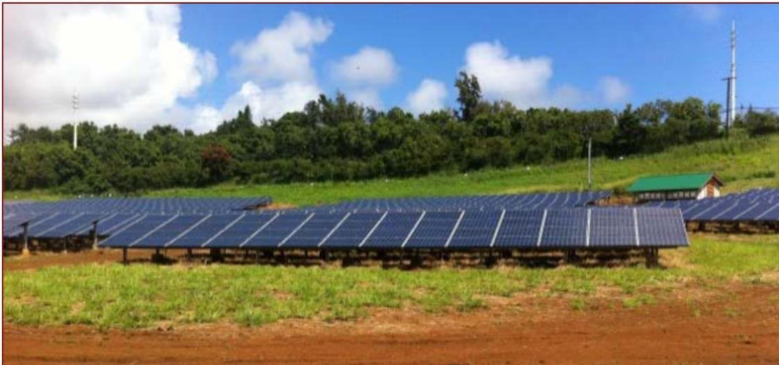
Figure 4-7: 1.2 MW<sub>DC</sub> Photovoltaic array on Kaua'i, Hawaii (Credit J. Keller, NREL)
