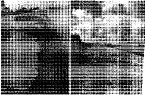
FAR LEFT: Post-flood cracking of the concrete at the Baton Rouge waterfront. LEFT: The same shot after stabilization with rock.
