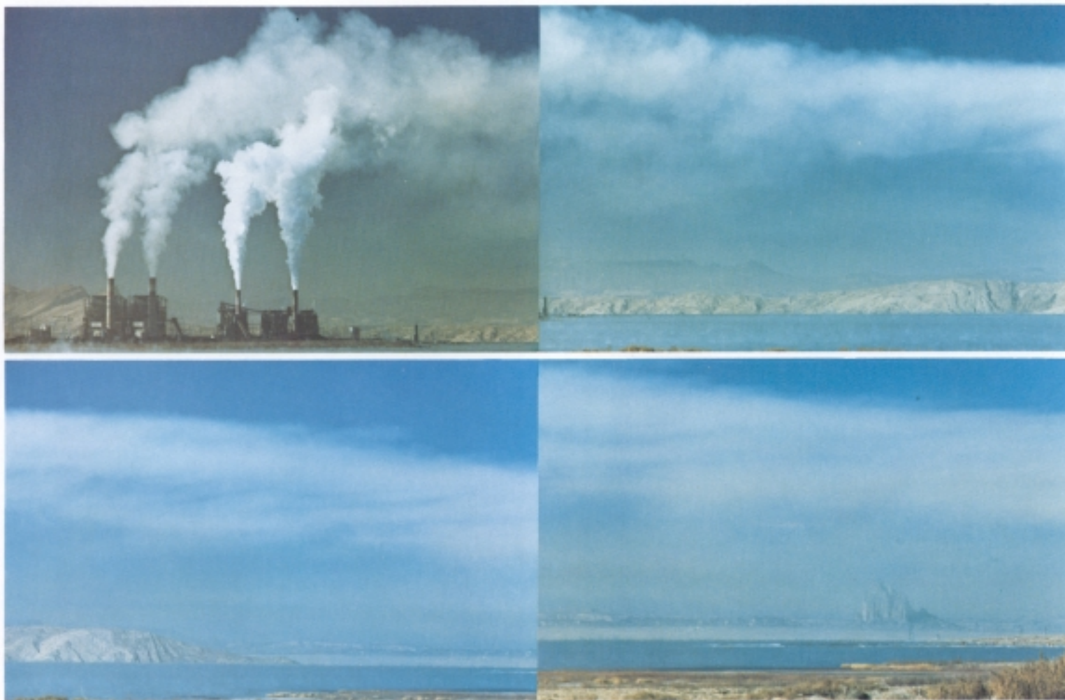
Figure 1-5. Near-source visibility impairment. Plume blight from particulate emissions extends downwind from the Four Corners Power Plant in New Mexico. As the plume mixes to ground level, the visibility of distant terrain features is degraded (Anderson, 1979).
