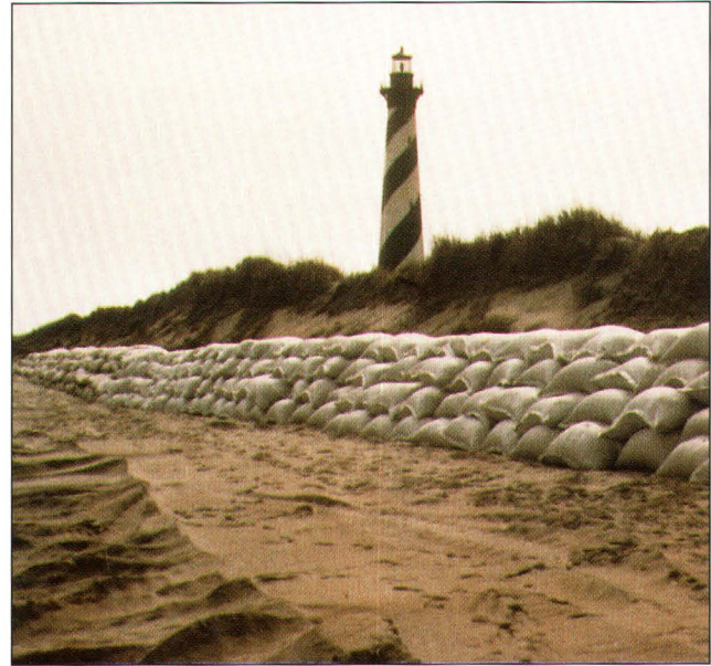
Figure 64. Sandbag seawall which was constructed at the base of the Cape Hatteras lighthouse. This structure was destroyed by wave action soon after it was completed. (Source: R. Dolan.)
