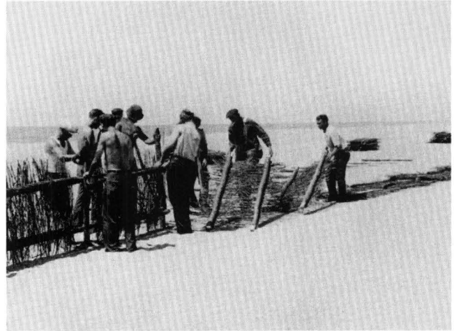
Figure 46. Sand fencing in 1936 to build barrier dunes along Hatteras Island. (Source: National Park Service.)
