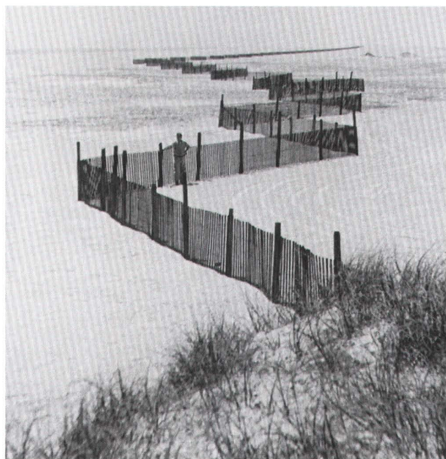
Figure 57. Sand fencing on Ocracoke Island. (Source: National Park Service.)
