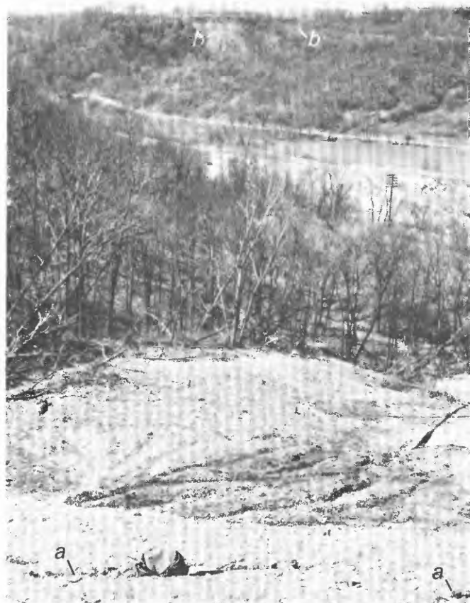
FIGURE 5.—Slides originating from regraded spoil-bank surface. Cracks ( a ) above head scarp indicate future retrogressive development. Slides in background ( b ) are similar to slide in foreground.
