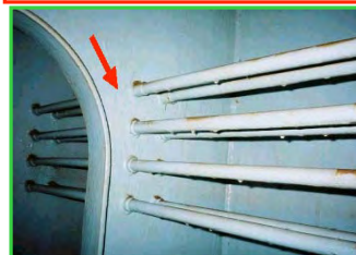
USS Ogden new technology tank coatings after 6 years
