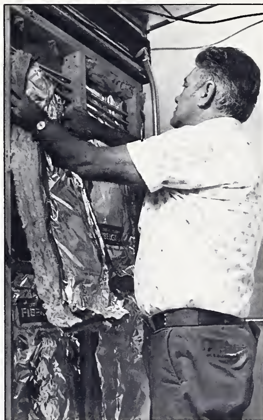
Adding insulation to check energy savings.
