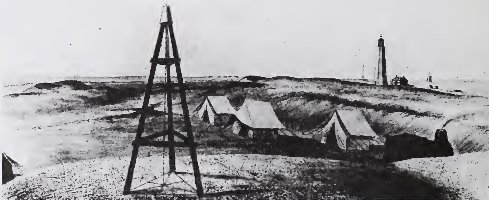
West Base station, above, showing the initial point of survey on Long Island, N. Y., and the survey camp of 1838.
