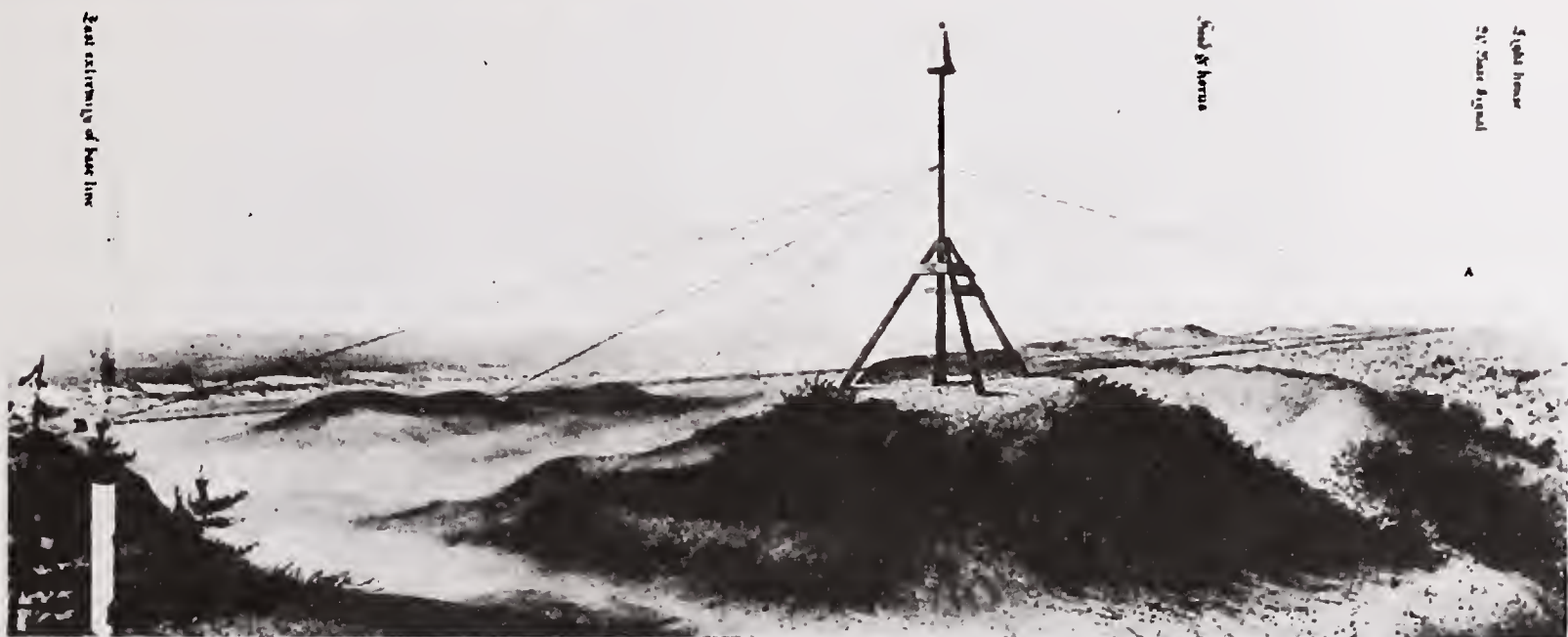
East Base of the original permanent base line laid out on Staten Island to initiate the primary arc of triangulation in 1839.
