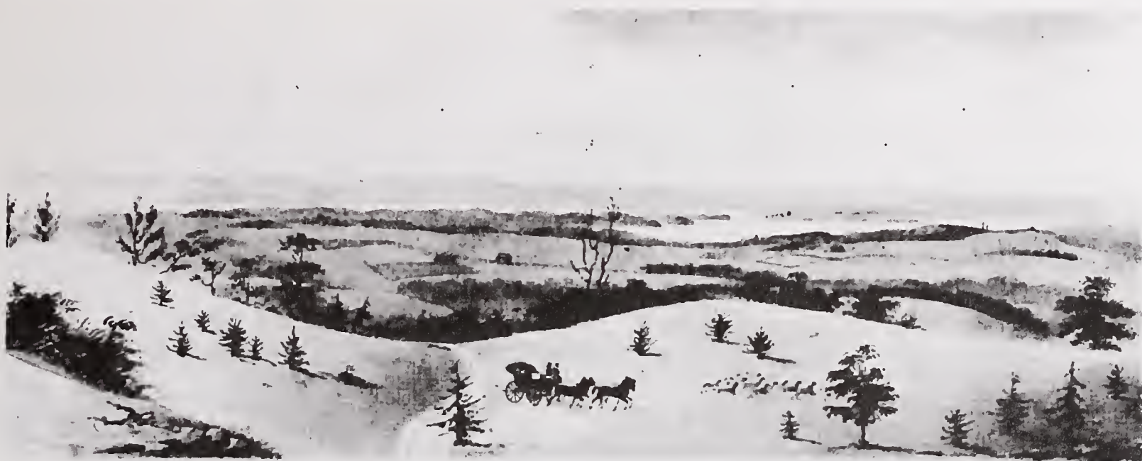
Southwesterly view from Harrow, N. Y., 1838, with Hassler's carriage and Great Theodolite, approaching the hilltop station.
