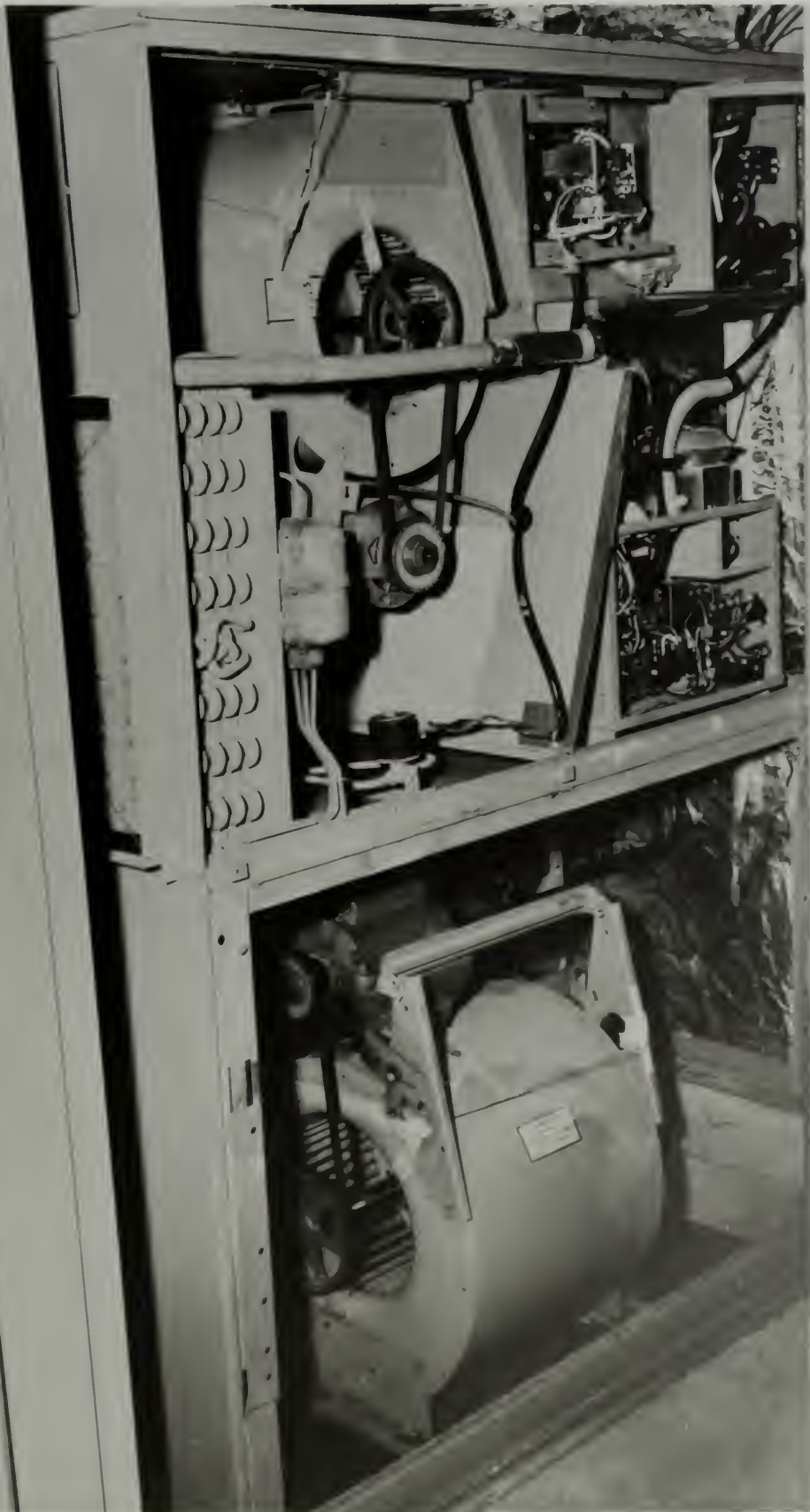
Fig. 17. View of typical unitary heat pump with front panel removed, Columbus AFB
