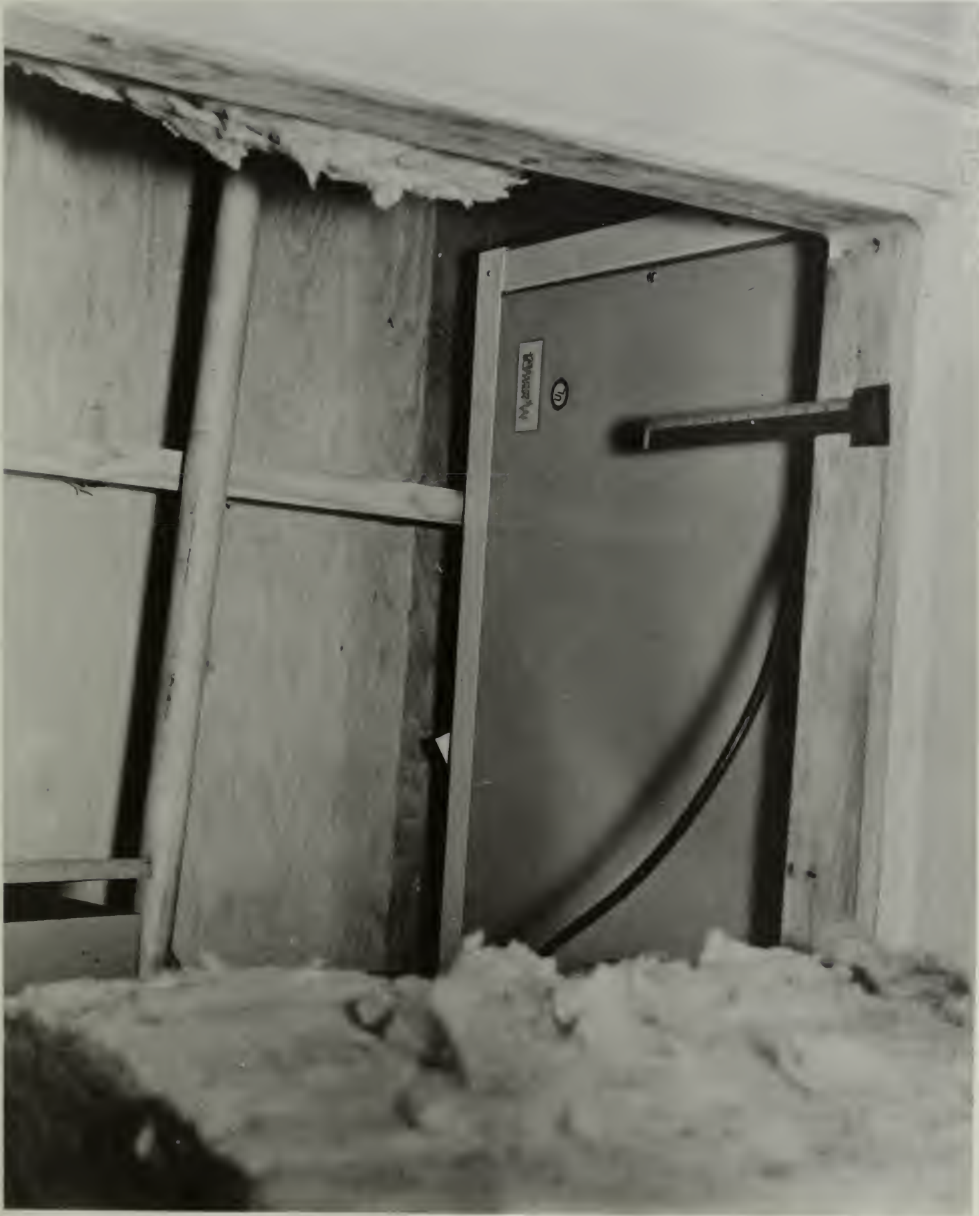
FIG. 13. Attic installation of indoor unit viewed through trap door, Seymour Johnson AFB
