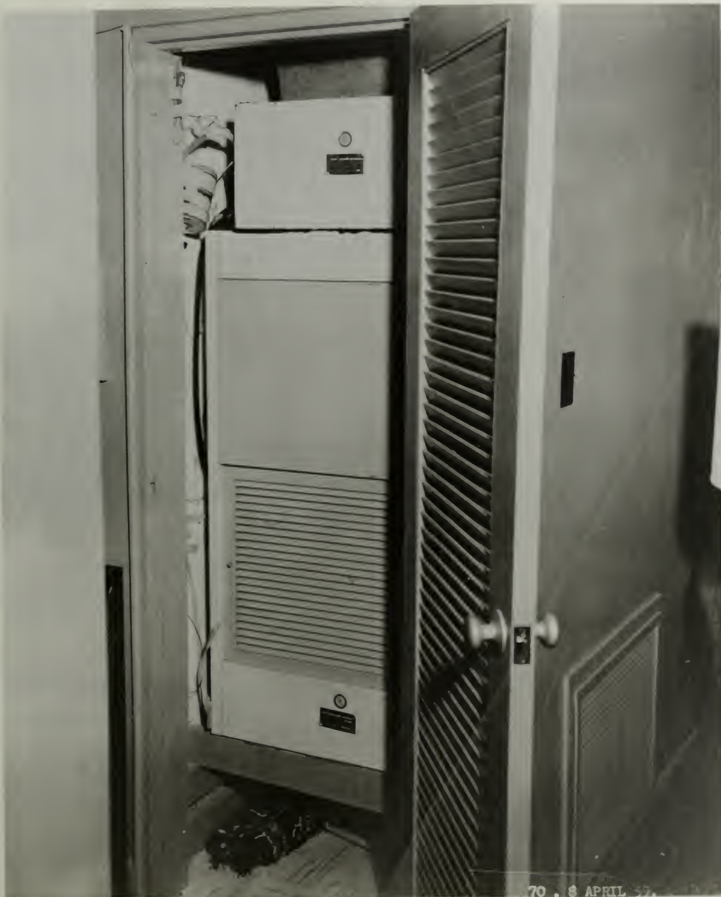
Fig. 14. Indoor unit in type E house viewed through closet door, Seymour Johnson AFB
