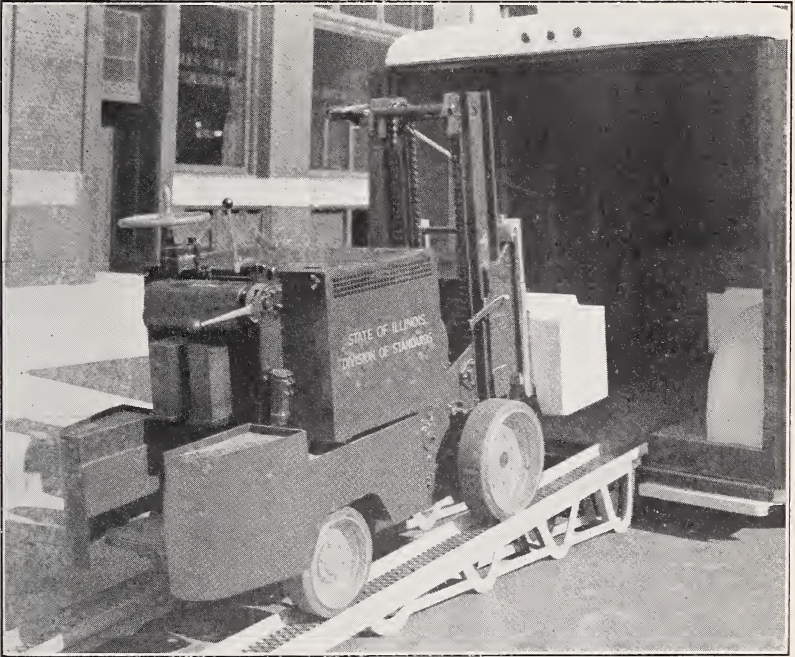
FIGURE 6.—Another view of Illinois equipment showing industrial truck, weights, and ramp.
