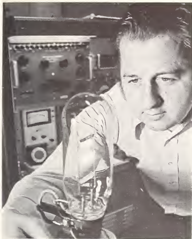
NBS standard of luminous intensity is used for industry calibration.
