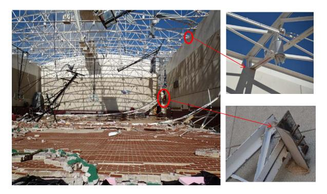
Figure 4. Example of photographic field data used in developing a failure hypothesis for the gymnasium at Joplin East Middle School. (Photo source: NIST)
