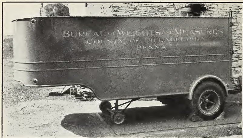
FIGURE 9.— Known-weight trailer portion of Philadelphia County, Pa., equipment spotted at one end of scale platform.
