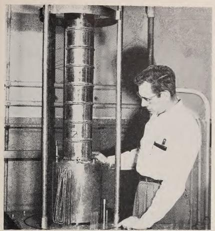
This distillation column, designed to investigate the separation of deuterium from ordinary hydrogen, is expected to provide valuable data for designers of large-scale equipment for producing heavy water (page 78).
