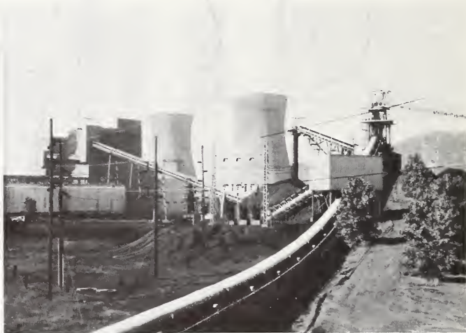
Figure D-3. Mitchell-Captina Power Plant with Cooling Towers and Conveyor from Sampling Building
